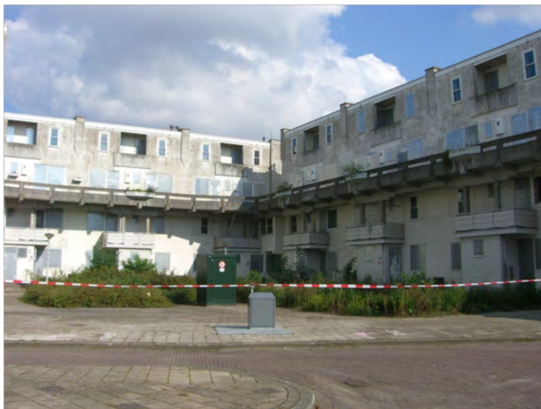
Figure 4. The complex in 2010, only twenty years after renovation and on the eve of the restoration.
