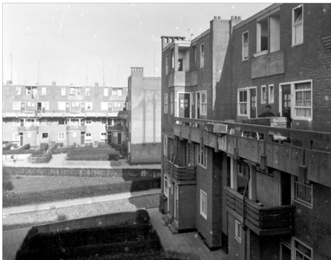
Figure 2. A detail of the gallery in 1924 (photo: MAR).
