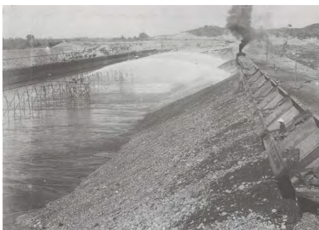
Figure 2. The construction work of the reservoir of Jianan Irrigation System. (Wu, 1998)
