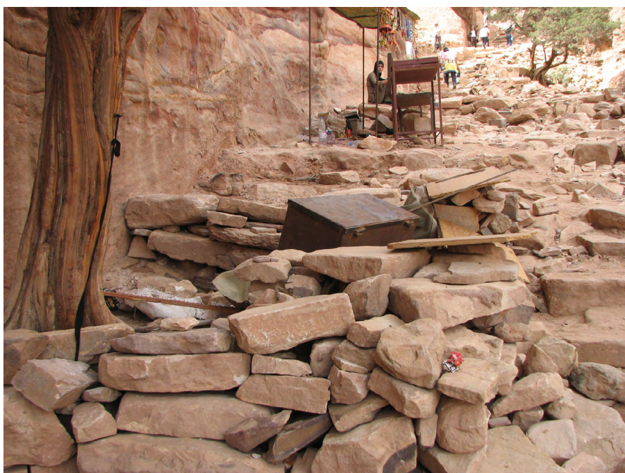
Figure 4: The long, processional stairway that leads to Ad-Dayr at Petra has been almost completely destroyed by the feet of donkeys carrying tourists. Photo by Douglas Comer.
