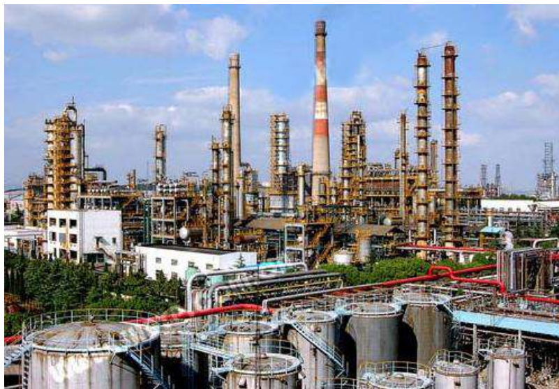
Illustration 4: Jinshan Petrochemical Plant
