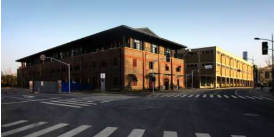
Illustration 6: Qinhuangdao Road Water Gate (East Wharf), Expo 2010 Shanghai.
