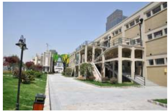
Illustration 8: Building A following protective restoration.
