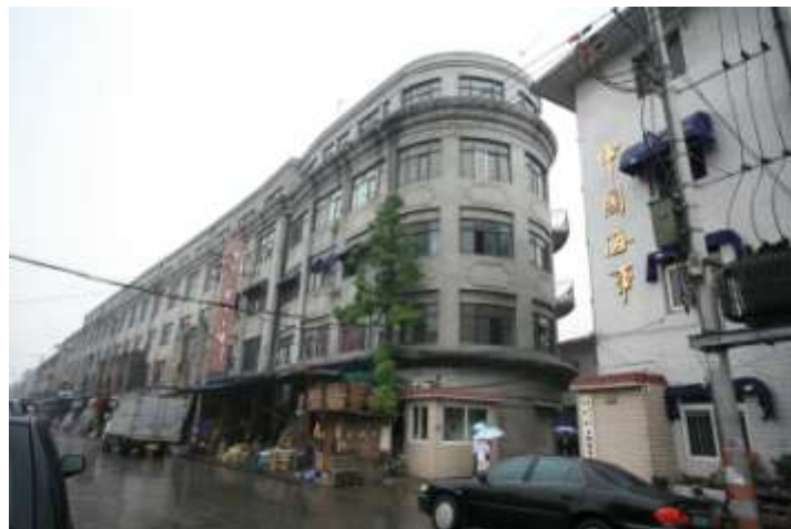
Illustration 3: Exterior and Façade of United Warehouse building
