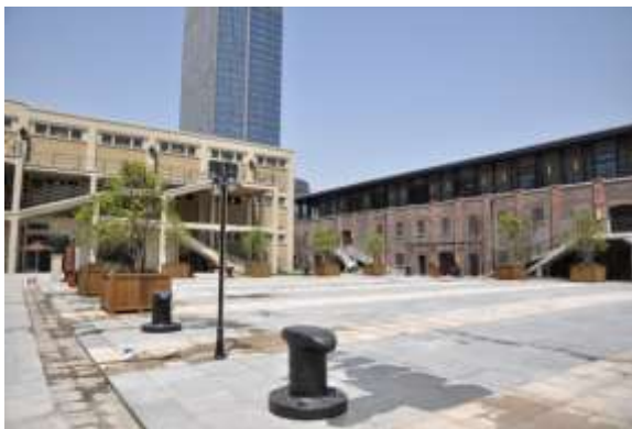
Illustration 7: Buildings A and B following protective restoration.
