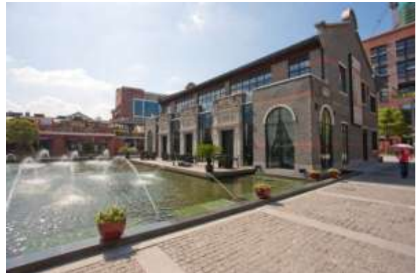
Illustration 6: Block scene of the South Bund after partial completion of redevelopment
