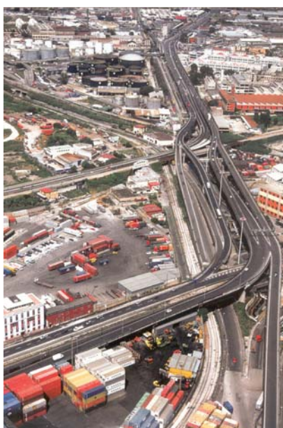
Figure 1 A big infrastructure junction near the harbour in the Eastern zone of Naples, Italy (photo Paolo De Stefano)
