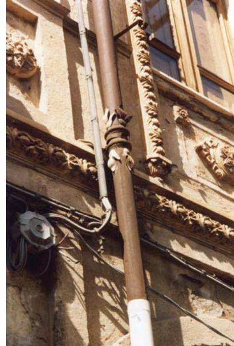
Quartu S. Elena (Italy), via Mori 129, detail of façade with obvious damages caused by telephone and power lines cables. (photo by G. Loddo).
