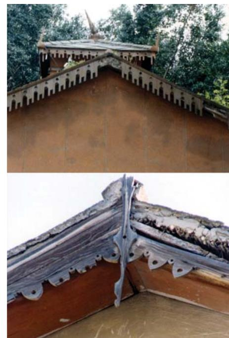
Bargeboards, Cagliari (Italy), top, wood and wrap metal modular elements, below, wood board element. (photo by G. Loddo).
