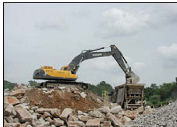
(Fig. 4) Rubble crushing.
