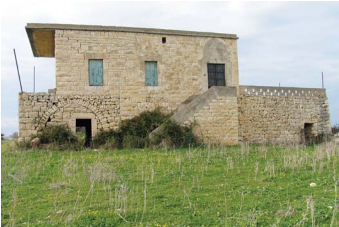
Simple rural house' in Ain Ikrin, with the addition of a 'gallery'. Six visible phases. Until the replacement of the earth roof with a concrete one and the obstruction of the gallery with concrete. (Photo by author, 2006)
