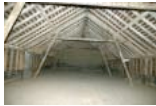
Figure 16. Upper loft in stables, minimal impact.
