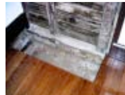
Figure 21. Interior, original earth floor and walls exposed.
