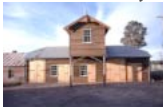
Figure 10. Reinstated façade with upper-storey.
