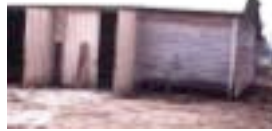
Figure 8. Steel doors on former Creamery.
