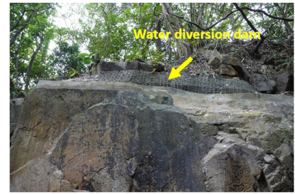
Figure 52. Water diversion dam above the rock carvings cannot drain away water effectively
