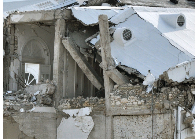
Figure 14. The 90-year-old National Palace in Port-au-Prince after the earthquake and partial demolition, revealing the reinforced concrete frame infilled with rubble stone. The steel reinforcing bars in the exterior portions of the frame and poured concrete walls (visible on left side of left photo) were heavily corroded in this over 90 year old structure.
