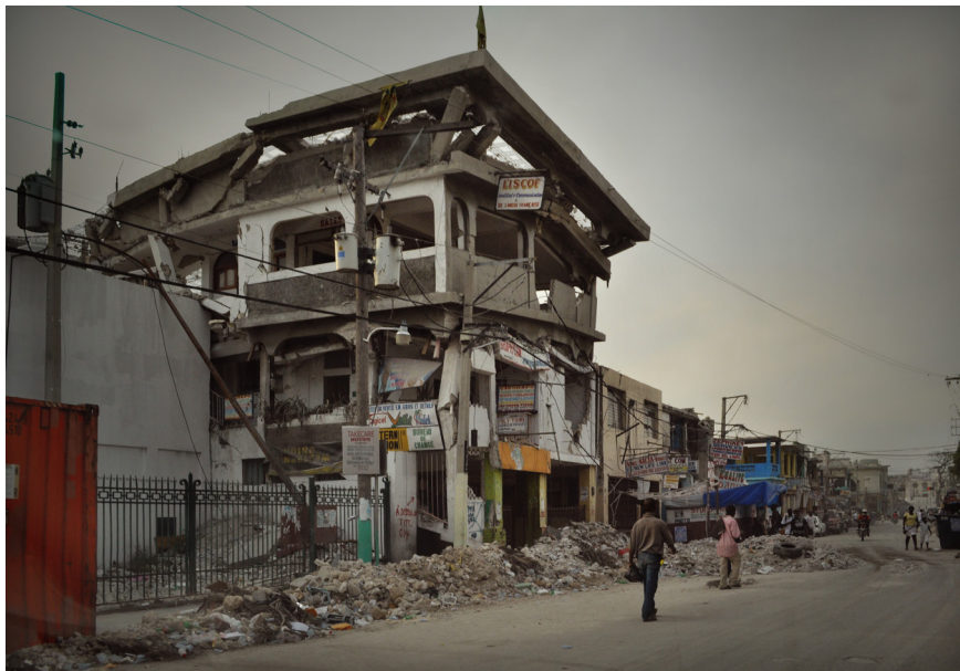
Figure 11. A downtown commercial building in a near state of collapse, illustrating the brittle vulnerable nature of many of the formal, contractor-built reinforced concrete buildings in Port-au-Prince. Many buildings of this type did pancake collapse, but as demonstrated by the buildings on either side that are still intact, everything did not fall down. Approximately 40% of the buildings in the central city were partially or totally collapsed; but of the remaining 60%, many suffered little damage 13
