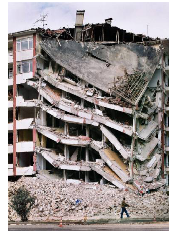
Figure 24. Building in Gölcük close to the one shown in Figure 23 collapsed by 1999 earthquake. The heavy masonry infill walls together with open (soft) ground floors were often contributors to such collapses.
