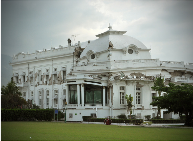
Figure 14. The 90-year-old National Palace in Port-au-Prince after the earthquake and partial demolition, revealing the reinforced concrete frame infilled with rubble stone. The steel reinforcing bars in the exterior portions of the frame and poured concrete walls (visible on left side of left photo) were heavily corroded in this over 90 year old structure.
