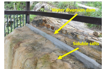
Figure 5. Leaching of soluble salts caused by an ineffectiveness of water diversion dam to intercept water flow
