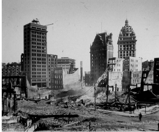
Figure 21. View of San Francisco after the 1906 earthquake and fire. The three tall buildings visible in this view were burned out by the fire that followed the earthquake, but all three were in good enough condition despite the earthquake and fire to be repaired. They are still standing to this day.
