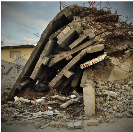
Figure 13. Left: Pancake collapse of a reinforced concrete building on the East side of Port-au-Prince. Pancake collapses of the heavy floors of multi-story RC buildings are particularly lethal and make it hard to extract the survivors. Right: A reinforced concrete building in Rikuzentakata Japan, swept onto its side and carried upstream by the March 10, 2011 earthquake and tsunami (Source: AFP/Getty)
