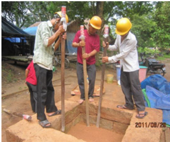
Figure 11. Rod compaction
