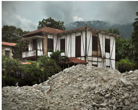
Figure 31. A Port-au-Prince house of colombage construction showing slight earthquake damage behind the rubble pile of a collapsed reinforced concrete building
