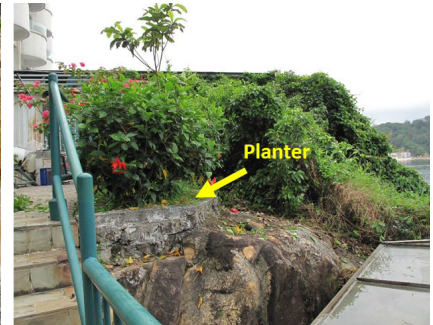
Figure 37. Planter above the rock carvings causes water seepage
