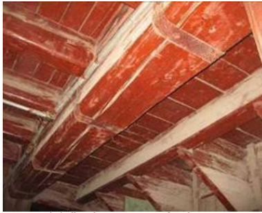
(a) flat iron straps for beam
