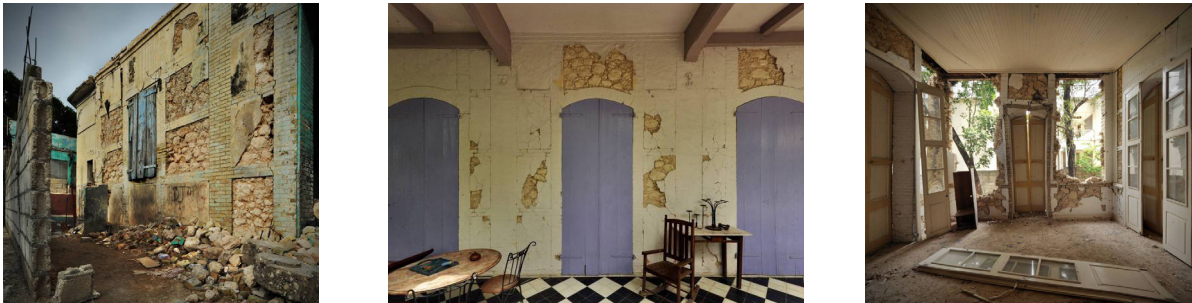
Figure 10. Brick and empaneled rubble stone construction, as is typically found in many of the Port-au-Prince ‘Gingerbread’ Houses from the late 19th century, showing different levels of damage from onset, to collapse of the rubble panels. Surprisingly few houses with this construction collapsed overall, despite the weakness and vulnerability to earthquake shaking of this construction – a further verification that the intensity did not exceed MMI-VII at these Port-au-Prince sites.
