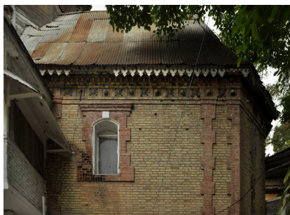
Figure 9. The unreinforced brick masonry of Hotel Oloffson, Port-au-Prince after the earthquake
