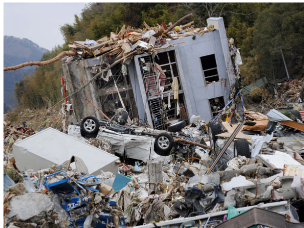
Figure 13. Left: Pancake collapse of a reinforced concrete building on the East side of Port-au-Prince. Pancake collapses of the heavy floors of multi-story RC buildings are particularly lethal and make it hard to extract the survivors. Right: A reinforced concrete building in Rikuzentakata Japan, swept onto its side and carried upstream by the March 10, 2011 earthquake and tsunami (Source: AFP/Getty)
