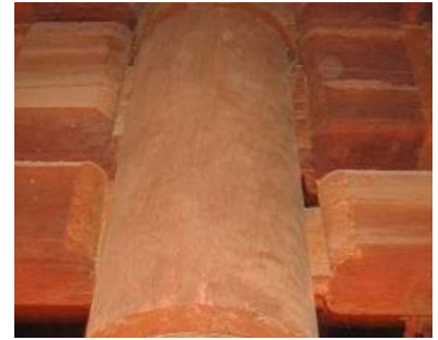
(c) tenon pulled out of mortise
