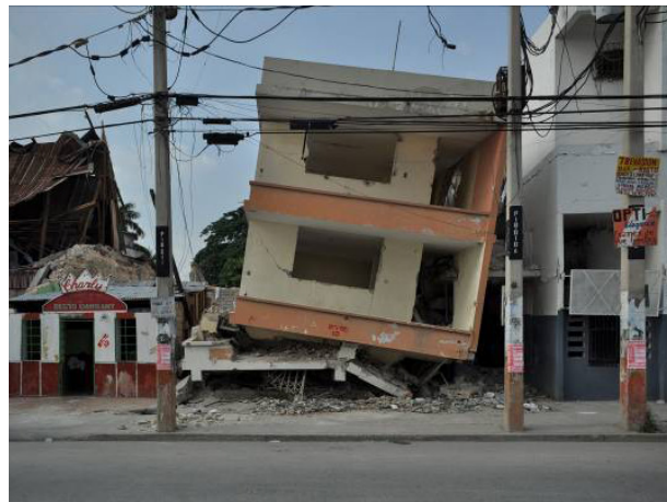
Figure 26. A formerly four story building in Port-au-Prince showing weak story collapse
