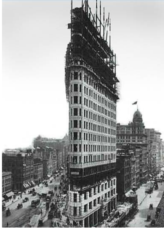
Figure 20. Flatiron Building in New York City under construction in 1902 showing the heavy stone masonry façade resting on the steel frame. The upper walls are constructed separately probably to ensure the weight is bearing on the frame rather than the lower masonry walls.
