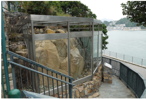
Figure 35. Glass enclosure creates a micro-climate which disturbs the equilibrium that had long been existed between the rock carvings and the natural environment as well as speed up the weathering process indirectly
