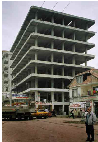
Figure 23. Building under construction in Gölcük, Turkey shown after the 1999 earthquake. Because the masonry infill walls had not yet been installed, frame action was able to occur, and thus the building was not collapsed by the earthquake.
