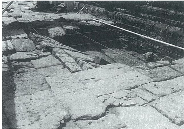
Figure 5. Damaged Pavement 60 years after archaeological excavation/backfilling (Source: JSA 2001)
