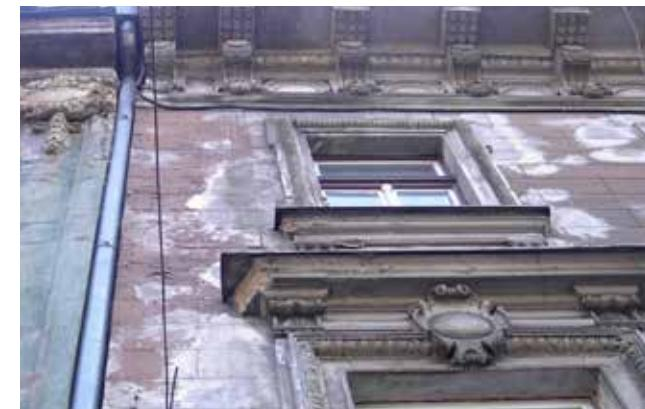
**Illustration 3.** Façade of the structure in Titova Street . Condition before the restoration and conservation design was compiled. Damage of the painted layer and mortar surfaces caused by increased humidity and decorative plastic art damage
