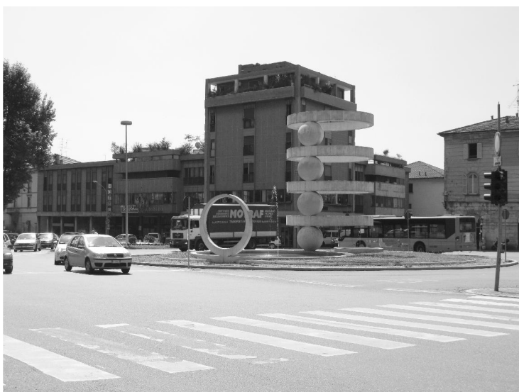
Fig. 1 Picture of the Camerlata Fountain
