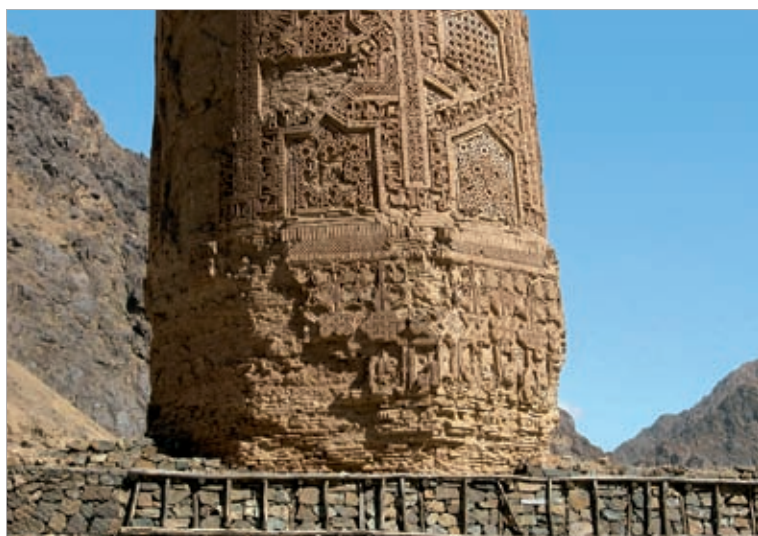
Fig.2 | Repair work on the damaged gabions around the Minaret of Jam (2003).
