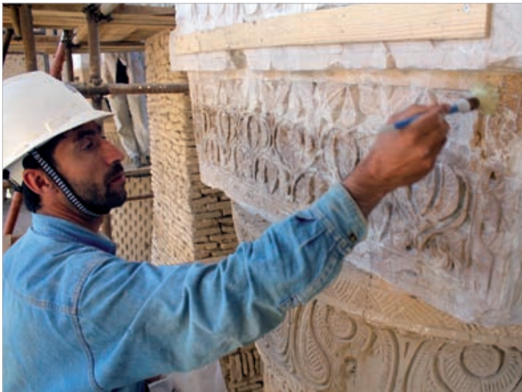
Fig.2 | Before structural consolidation work could commence, the exquisite stucco decoration adorning the surfaces of the building had to be stabilized and protected.
