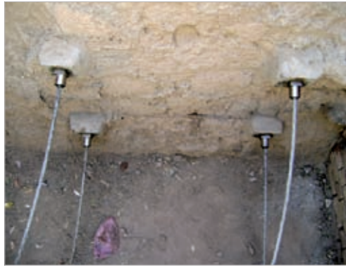
Fig. 20 | LEFT: Corroded stays of the Fifth Minaret (2010).
