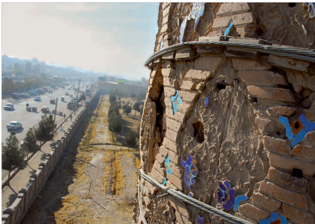
Fig.19 | Inspection of the stays supporting the Fifth Minaret (2010). PHOTO: © UNESCO/ C. MARGOTTINI
