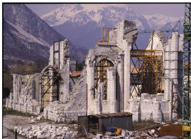
Fig 3, 3a. Images of the Duomo and the historical center of Venzone after the second earthquake of 15 September 1976 and after the shoring of the surviving walls of the Duomo.
