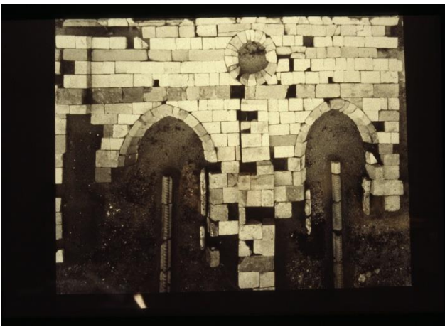
Fig 5, 5a. Zenith photo (R. Bertossi) and glimpse (F. Doglioni) of the stones of the Chapel of the Gonfalone recognized and reassembled on the ground
