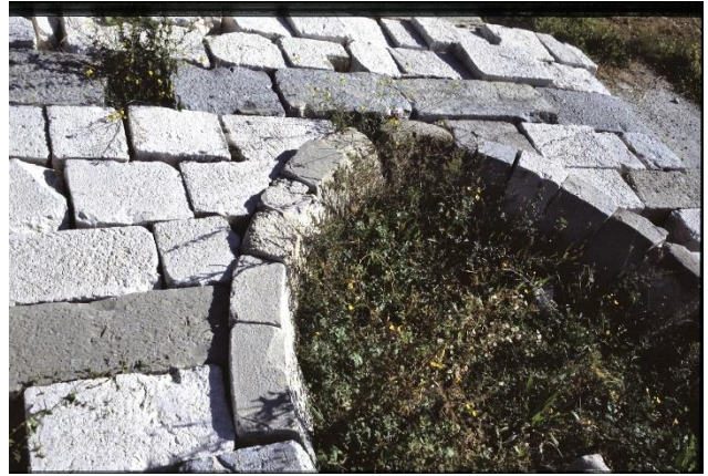
Fig., 5b, 5c. Detail of the recomposition chart of the stones of the Cappella del Gonfalone façade. The number indicates the symbol of the recognized stone and the placement direction. On the right, stones recomposed to the ground
