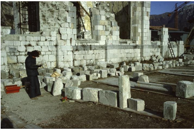
Fig. 4, 4a. The work of cataloging and recognizing the recovered stones. On the right, one of the large stone deposits.
