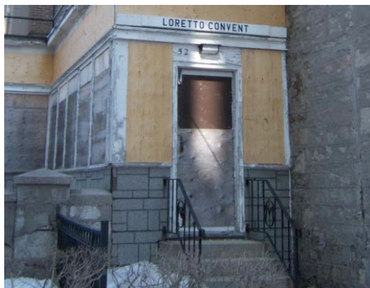
Figure 1. Loretto relief pointing & asphalt pattern
