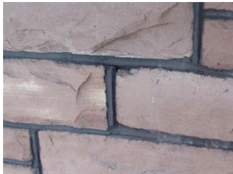
Figure 7. RCM, new overhung ridge joints
