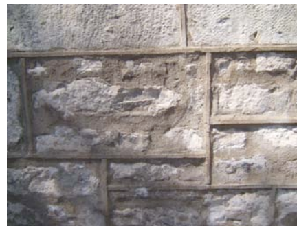
Figure 4. Detail of relief joints
