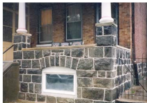
Figure 13. Cobweb ribbon joint
