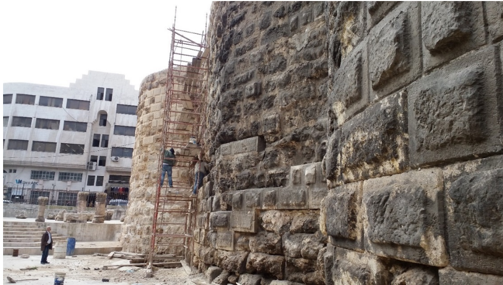
Fig.5- Consolidation works at the back side of the monument ©Authors.
