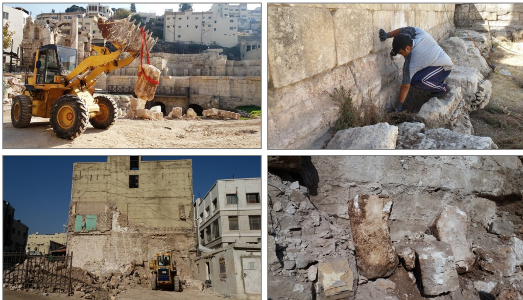
Figure 3– Cleaning process and preparation works at the site, ©Authors.
