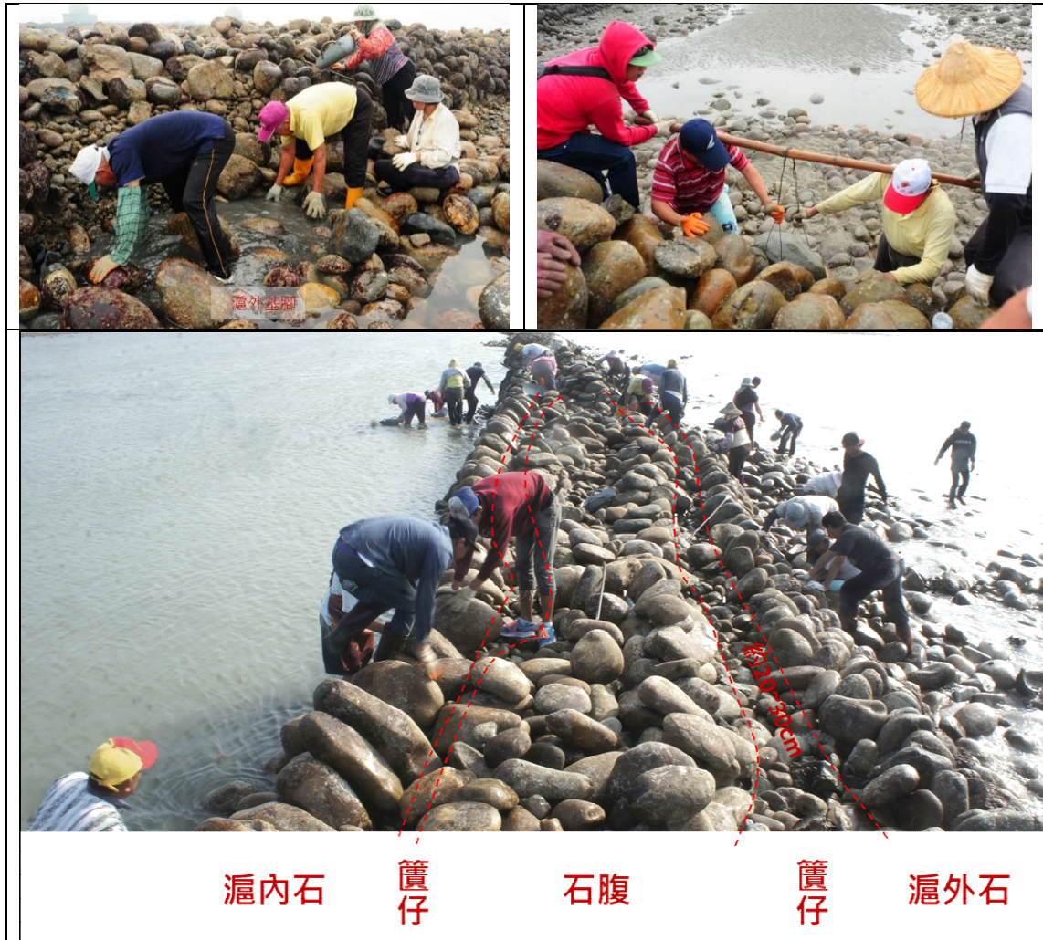
Fig.8- Cooperation of weirs construction
