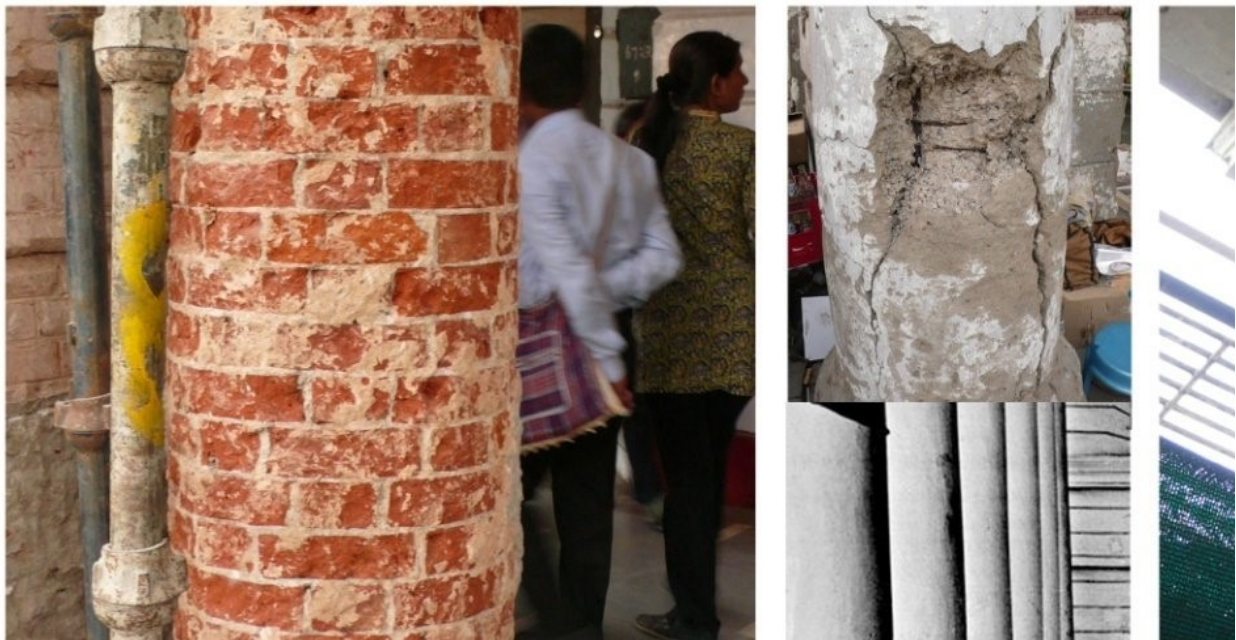
Fig.6- Lime plaster and mouldings replaced by Cement plaster
