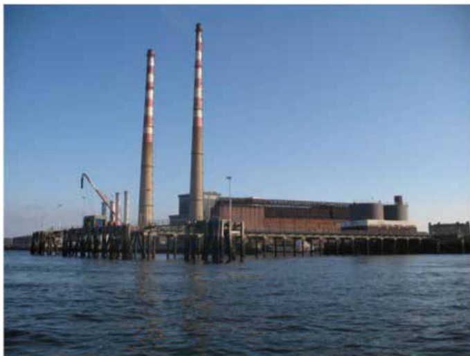
Fig. 5: Electricity Generating Stations, Dublin: The two tall chimneys are from the Poolbeg Station built 1965-1971. The low red-brick building on the right is the 1903 Pigeon House Station, and was an early pioneering example of three-phase electricity generation.
