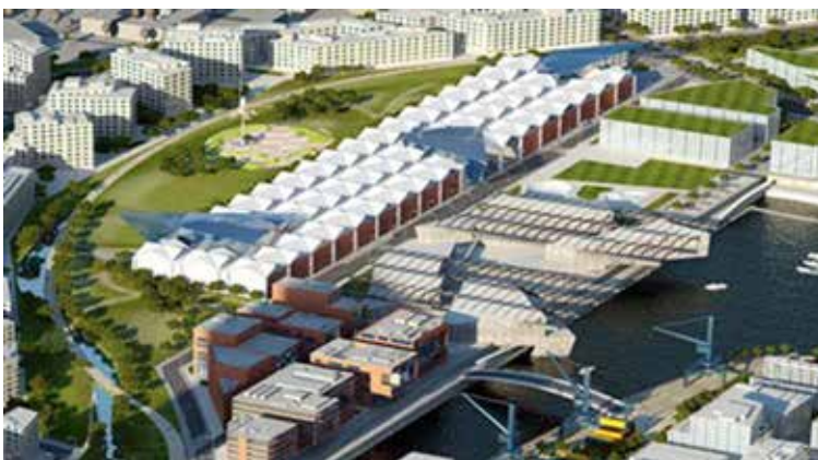
Fig. 3: Reconstruction of industrial heritage in Port of Belgrade. Source: http://www.lukabeograd.com .
