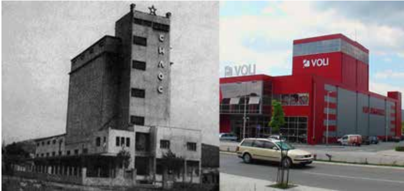
Fig. 2: The old silo in Niksic, 1935 – The new envelope and unsuccessful “rebranding” of the town landscape (Left photo by Enciklopedija Jugoslavije, tom 2. (1956), Zagreb: Leksikografski zavod FNRJ, p. 462; Right photo retrieved June 10, 2016, from http://www.ramel.me/page.php?cat=5 ).
