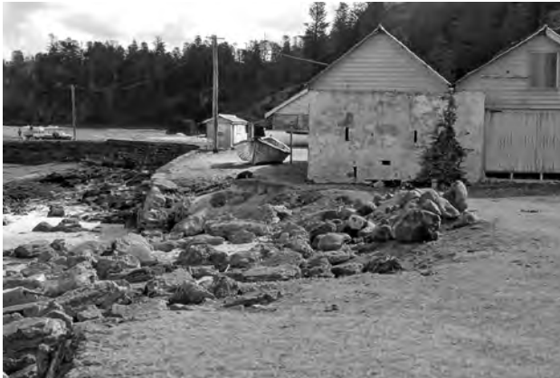
8. Breach in the sea wall at Kingston, Norfolk Island. JSK photograph 1978.
