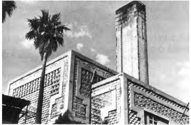
25. Reverberatory incinerator, Pymont, NSW, with applied patterns still intact. JSK photograph 1962.
