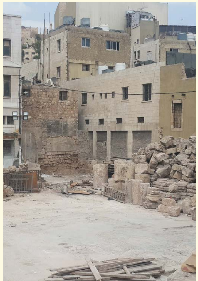
Fig. 107: The area after the removal of the barracks.
