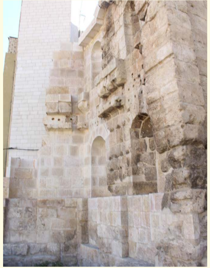
Figure 33 and 34: Eastern part before (left) and after (right) finishing the buttress construction
