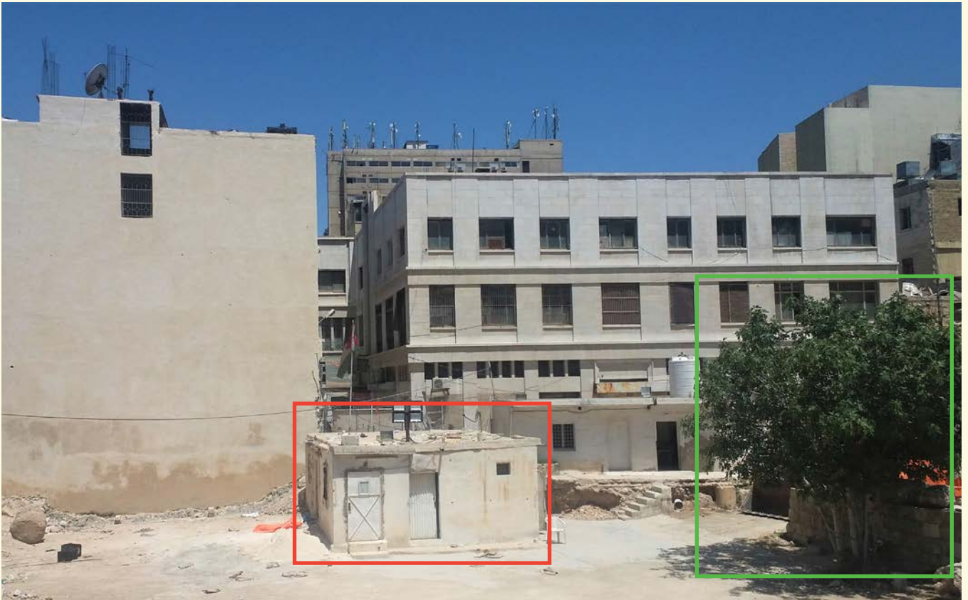
Fig. 108: The DOA temporary rooms and the fig tree before removal
