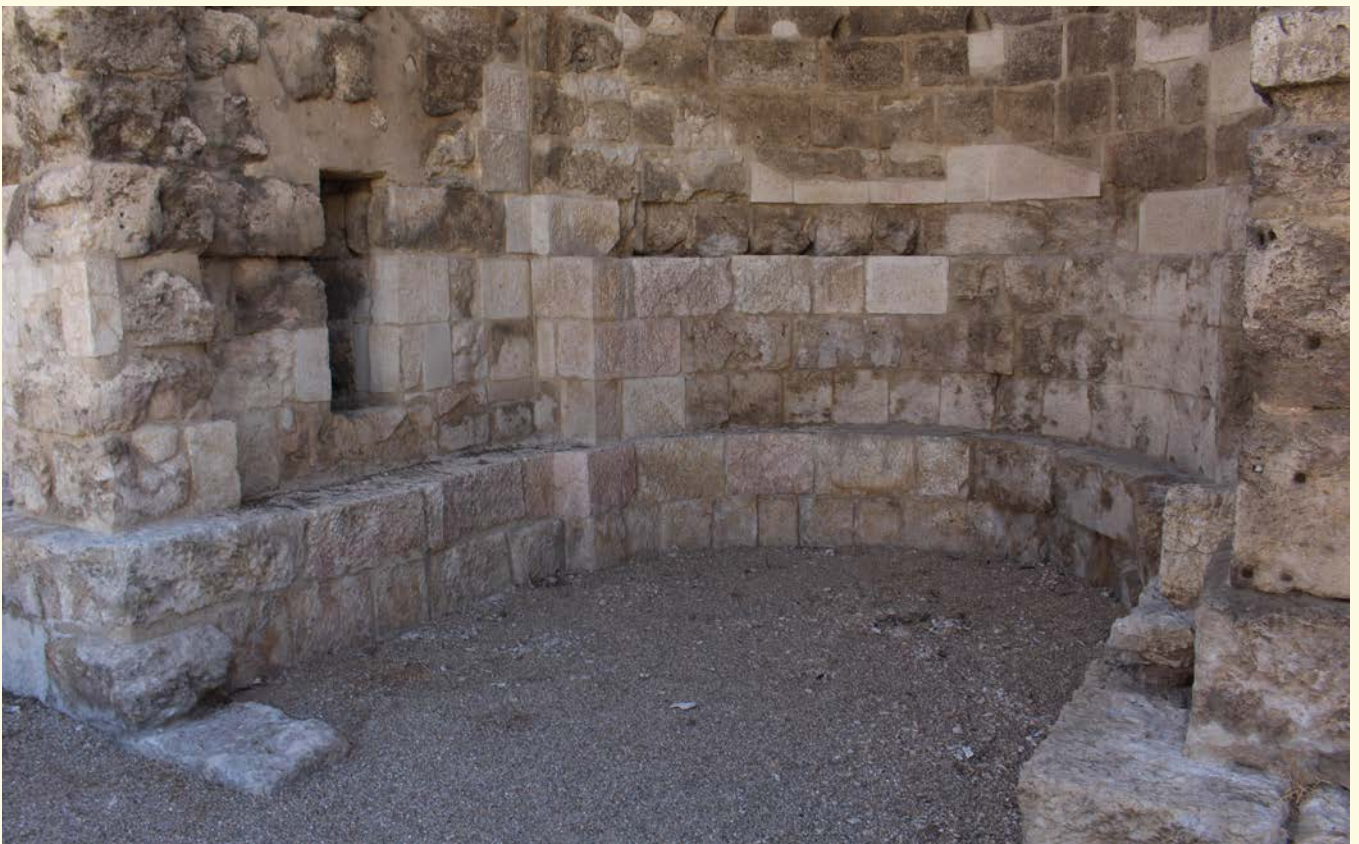
Fig. 114: Basin after end of project restoration and conservation and the basin covered with gravel
