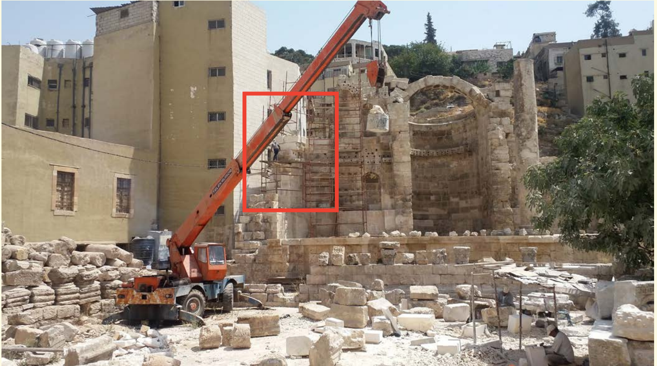
Figure 25: Reconstruction work at the area (A) as shown inside the red rectangle.
