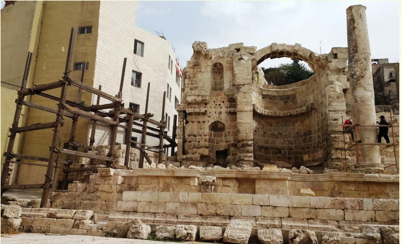
Figure 29: Eastern part before buttress construction
