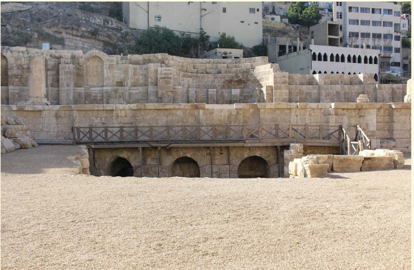
Fig. 132: Front façade with the new bridge extension at the end of the project with all restoration and conservation works concluded and the site ground covered with gravel
