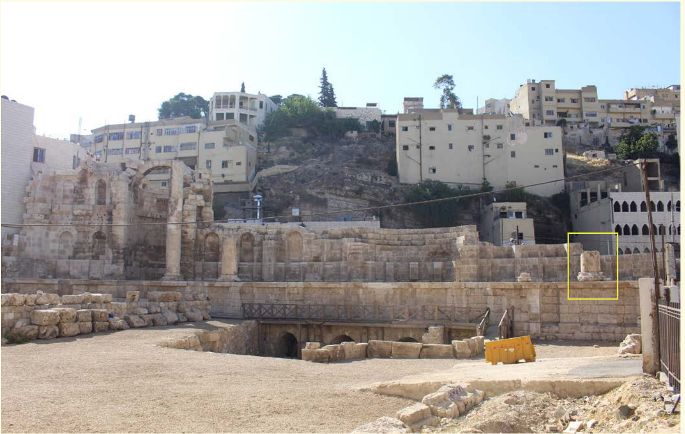
Figure 42: Reinstalling one of the columns into its proper location in the monument
