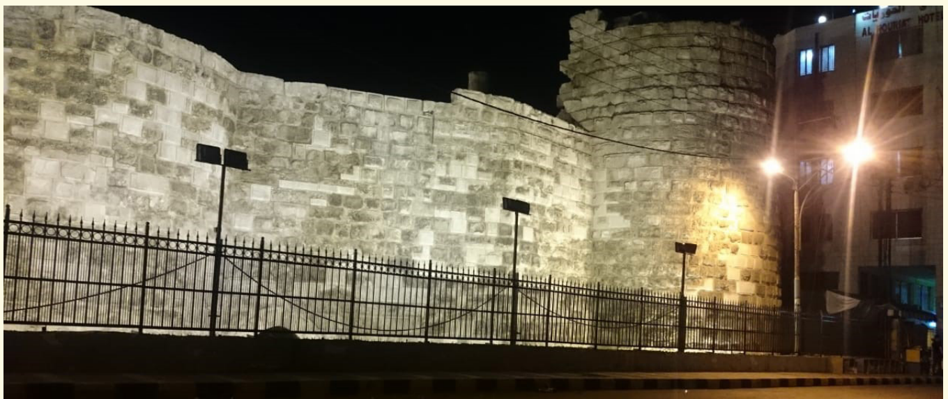
Fig. 119: The Nymphaeum with lights at night and with the new fence after installation.
