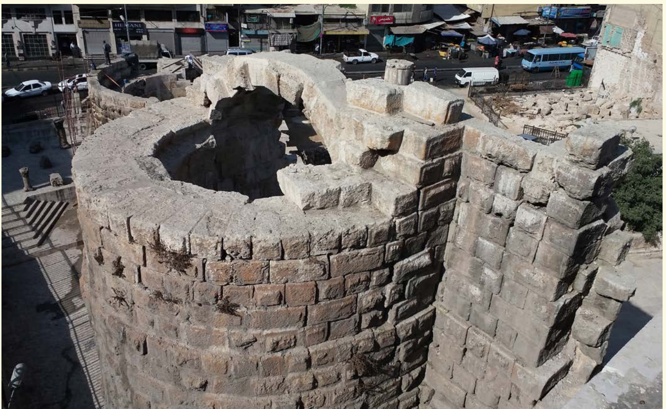
Fig.8: A view of the Nymphaeum from the nearby hotel during project implementation.
