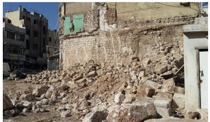
Fig.12: Removal of previous structures from the site.
