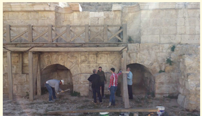
Fig. 130: The project team during the discussion of the bridge extension.
