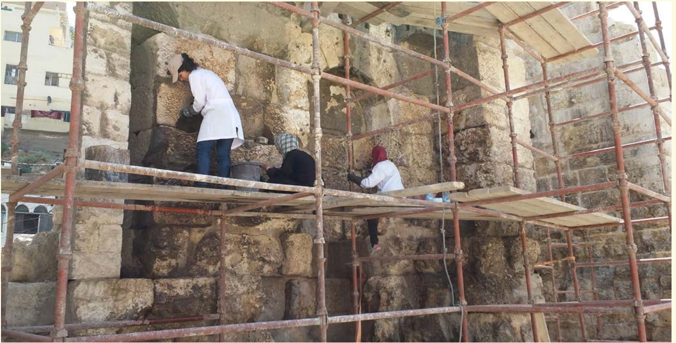
Fig. 103: Students working on façade cleaning
