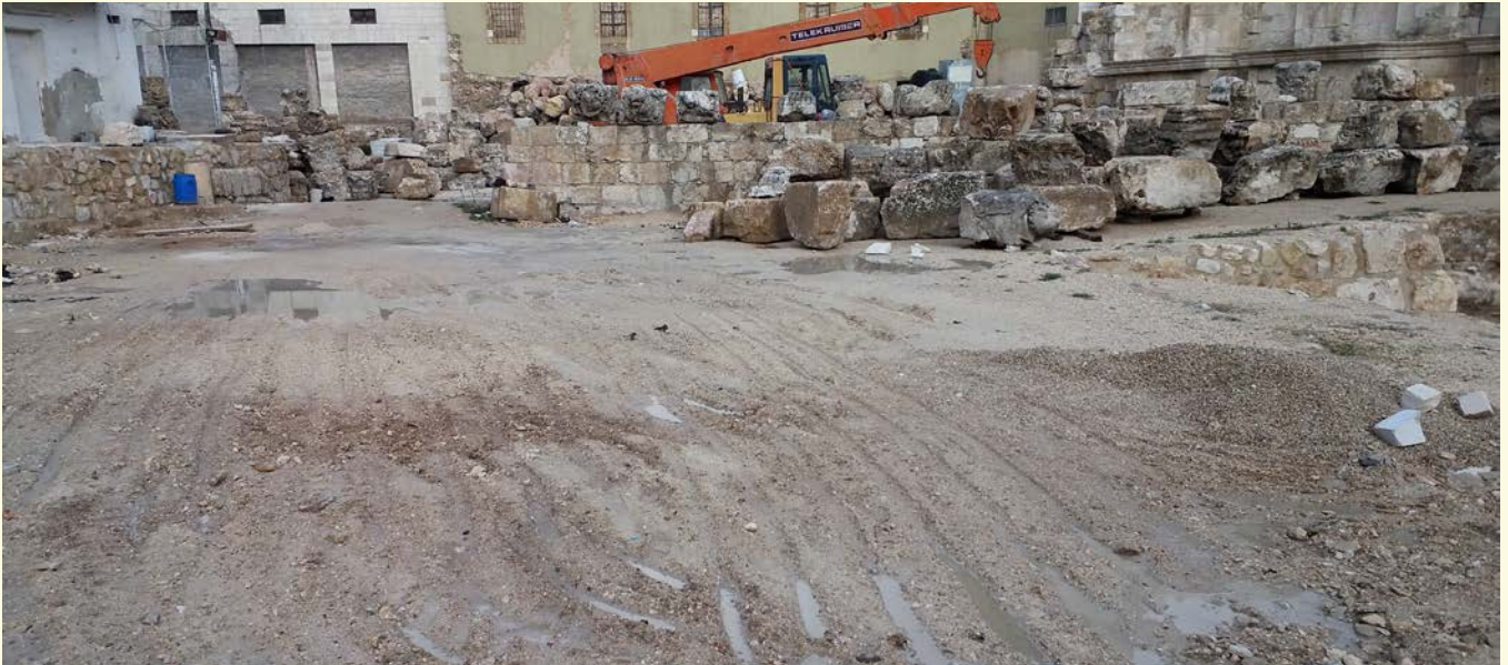
Fig. 111: Site during leveling and before ground was covered with gravel
