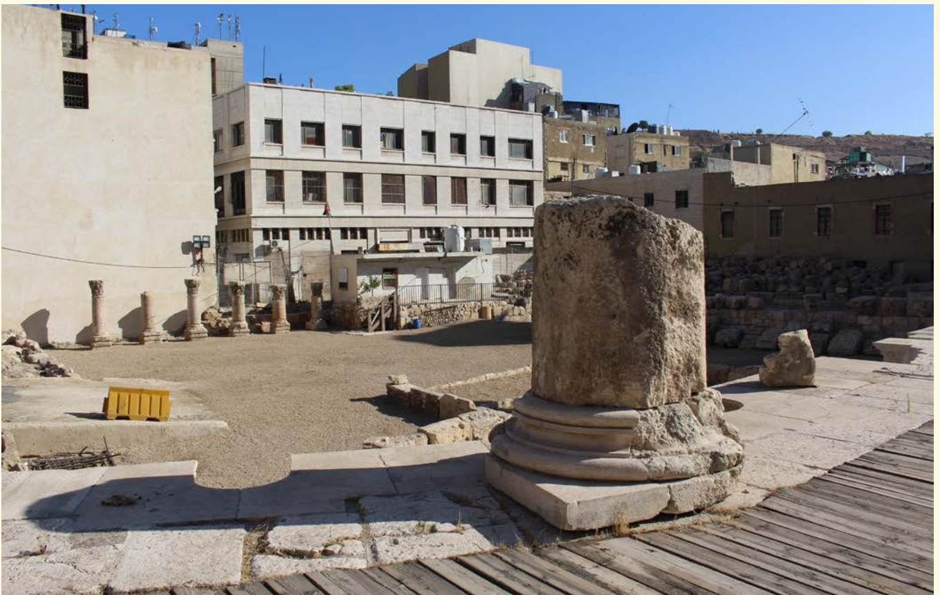
Figure 43: Reinstalling one of the columns into its proper location in the monument
