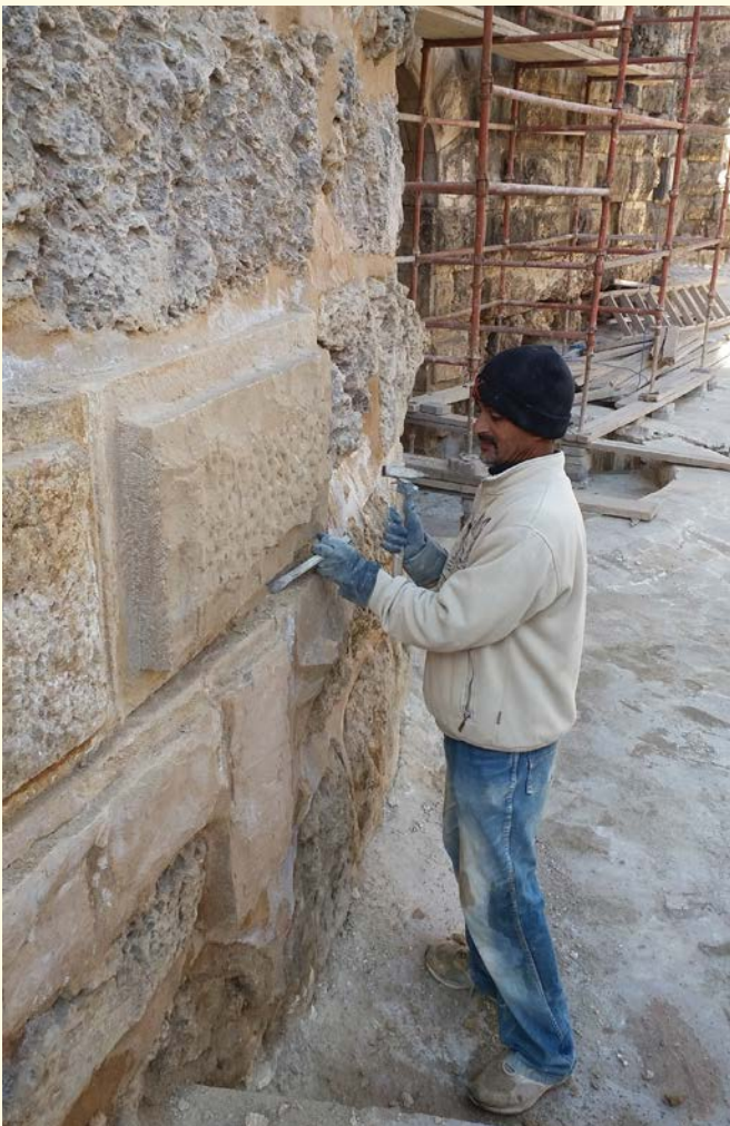
Fig 48: During consolidation at the rear façade
