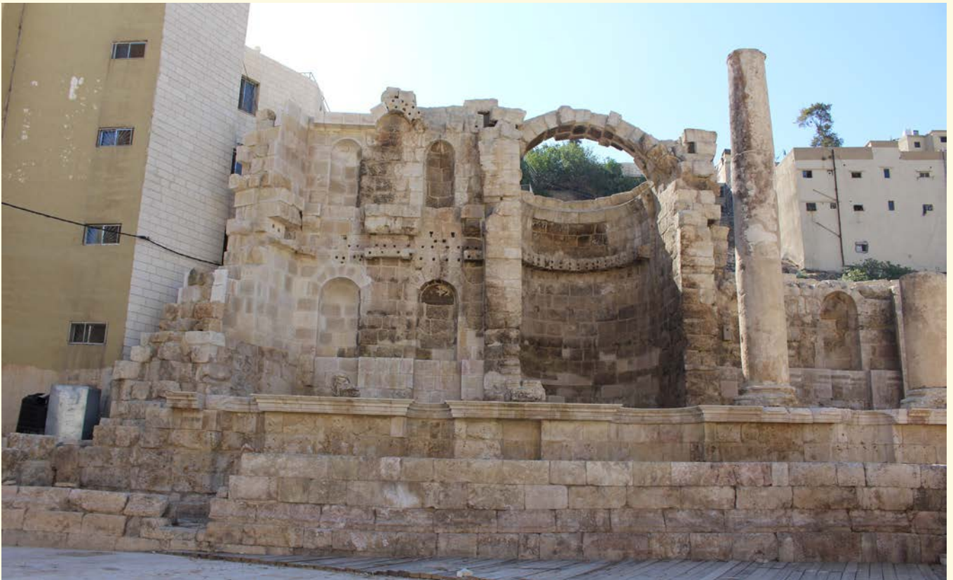
Figure 30: Eastern part after finishing the buttress construction
