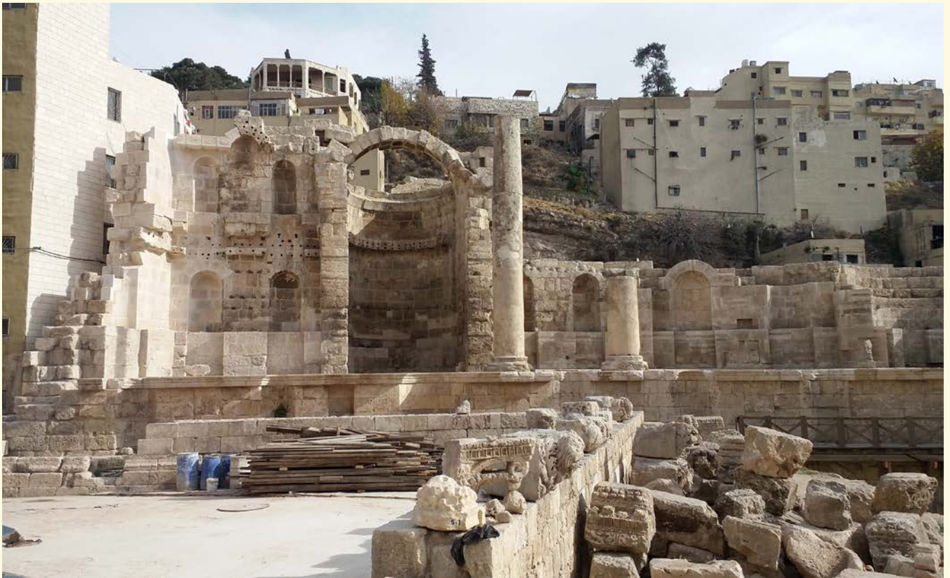
Figure 28: Buttress after finishing the construction work which highlight the success of the intervention as it enhanced the architectural interpretation of the monument and enhanced the stability of the structure.
