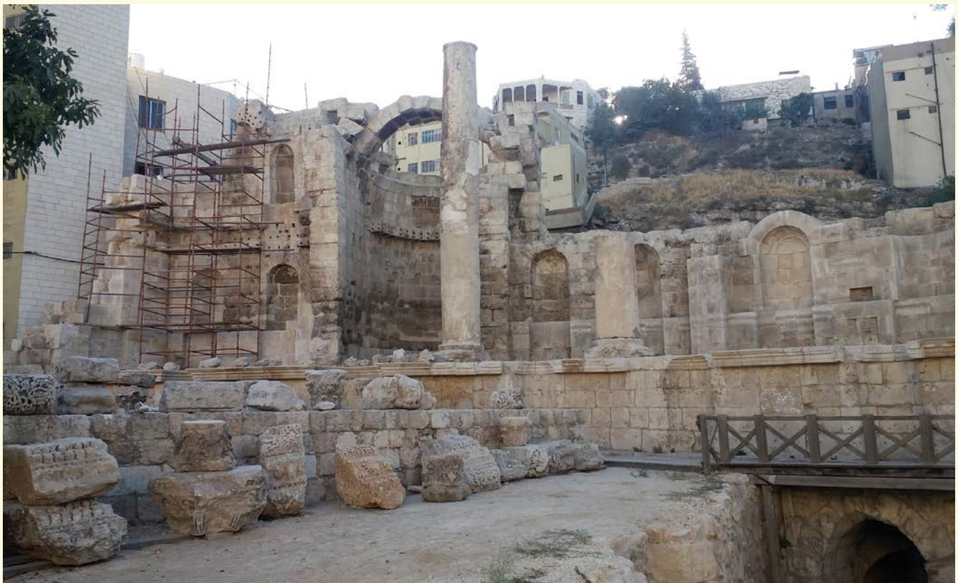
Figure 26: Buttress construction in progress
