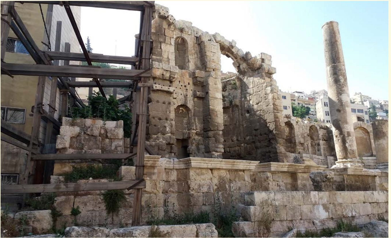
Figure 31: Eastern part before buttress construction
