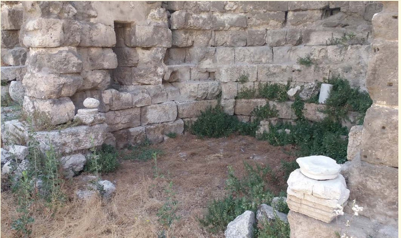
Fig. 113: Basin before starting the project interventions
