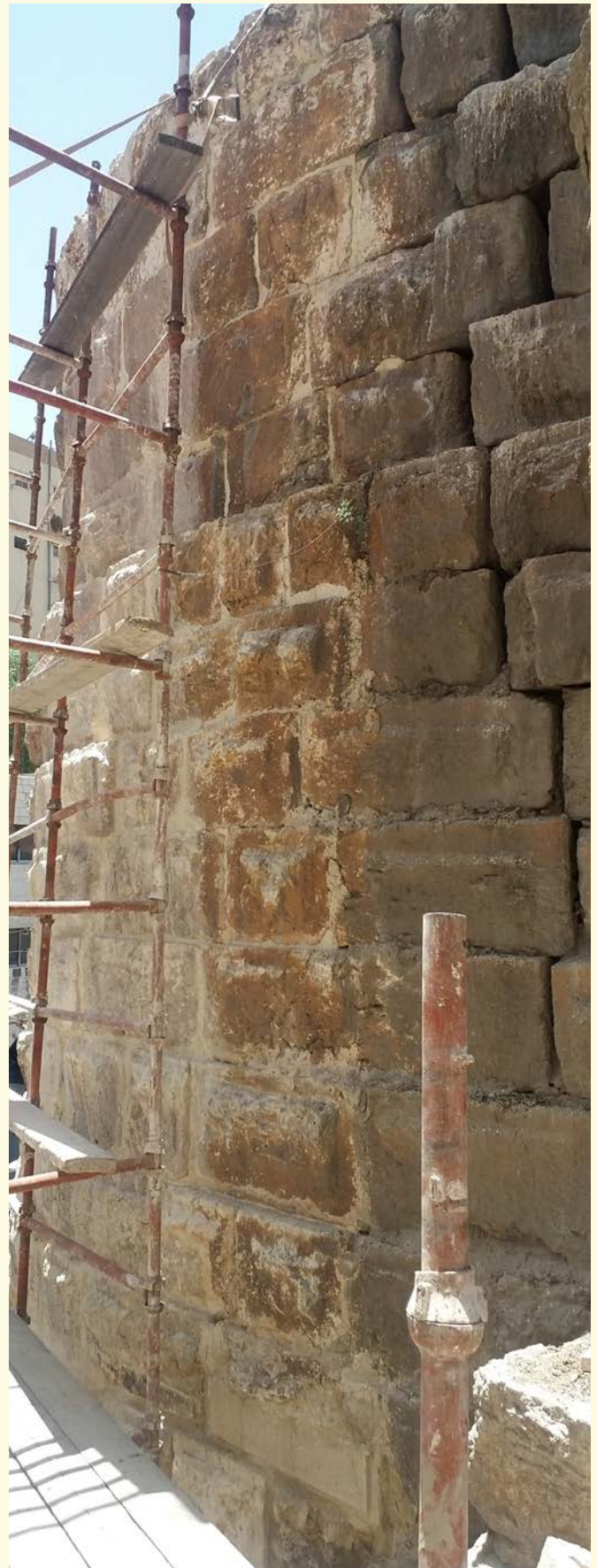
Fig. 13: During the cleaning stage of the site with a clear view of a major crack.
