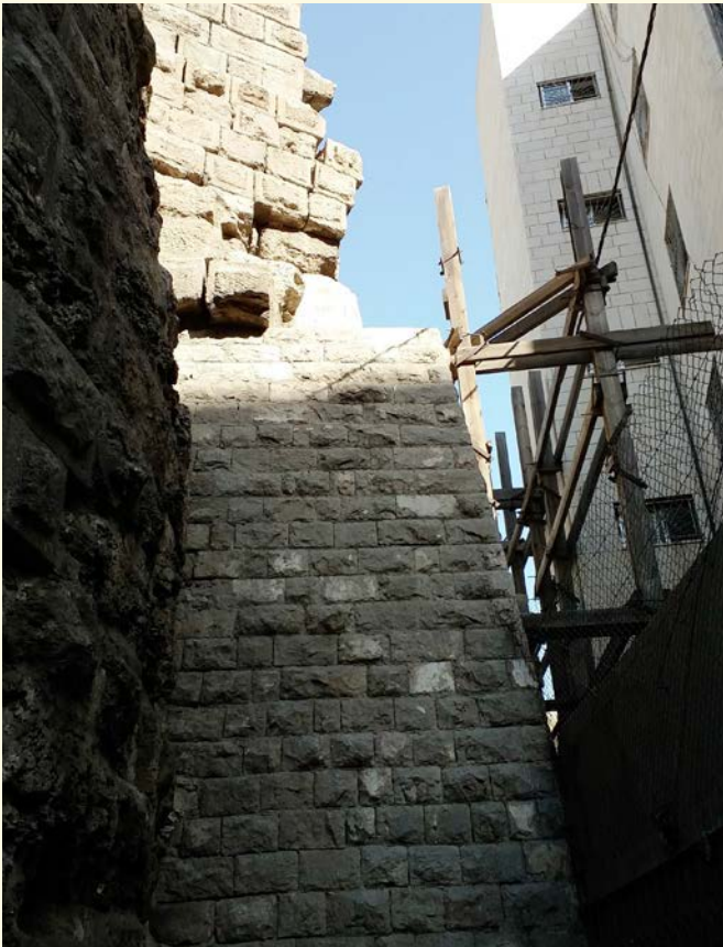
Figure 35 and 36: Rear of Eastern part before (left) and after (right) finishing the buttress construction
