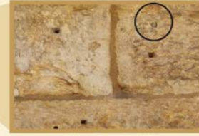
شكل (2): بقايا الإسمن الرخامي والحاسي Figure (2): Remains of the marble and copper anchor
