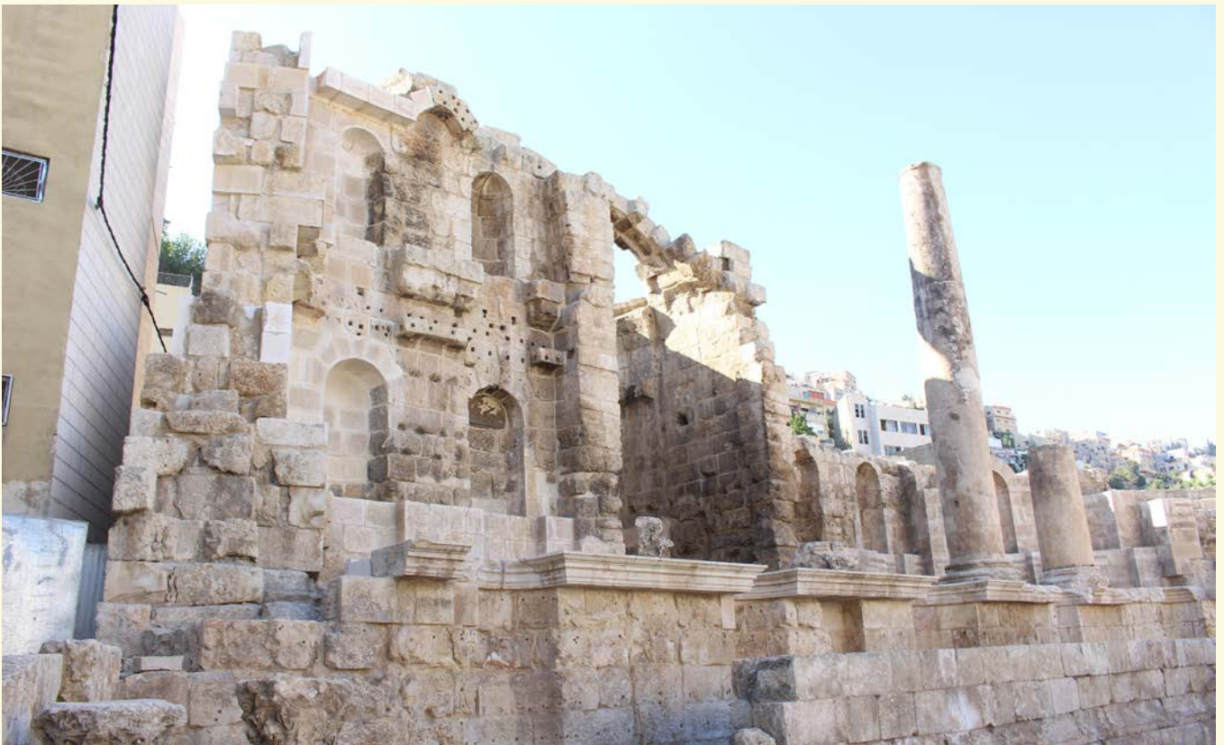
Figure 32: Eastern part after finishing the buttress construction
