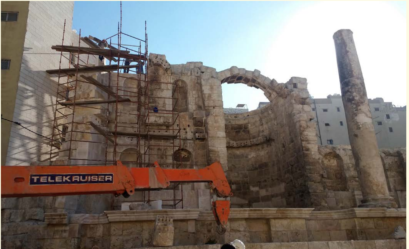
Figure 27: Close-up photo of butress construction using scaffolding system and crane
