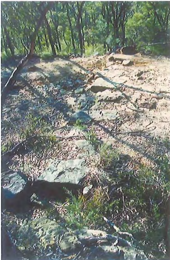
Figure 4-30: Capping stones over road culvert, between Devine's Hill and Finch's Line. (from OGNR Conservation Management Plan, NPWS, 1999. Photo Jeff Betteridge).
