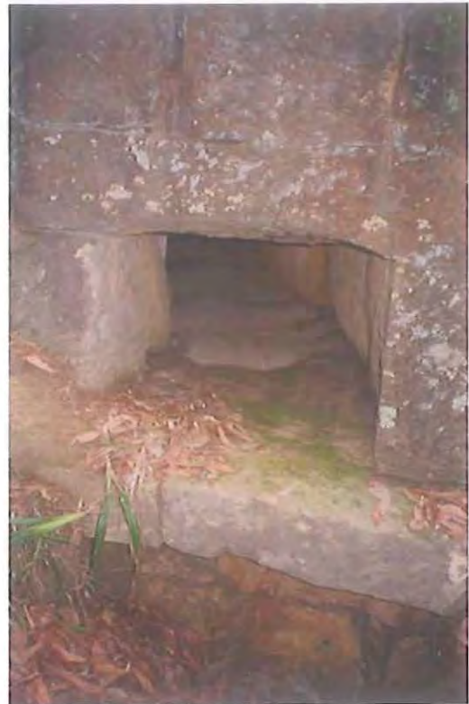
Figure 4-27: Stone culvert in base of road formation. (Photo: Lesley Walker)
