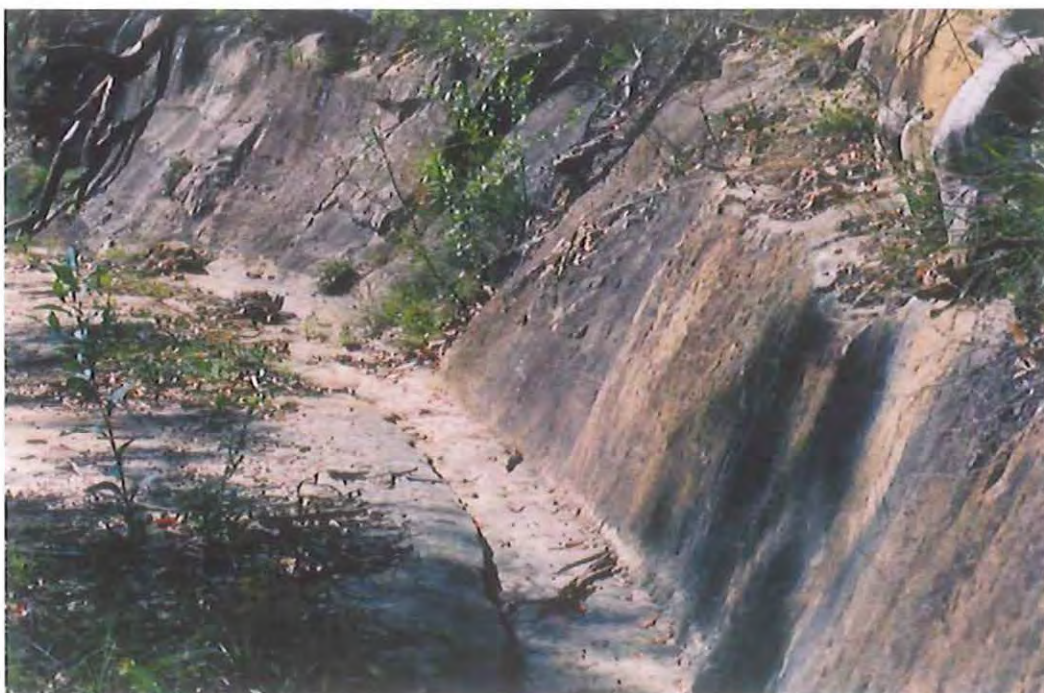
Figure 4-25: Side drain picked into rock, between Western Commission Track and Ten Mile Hollow. (Photo: Ingereth Macfarlane)
