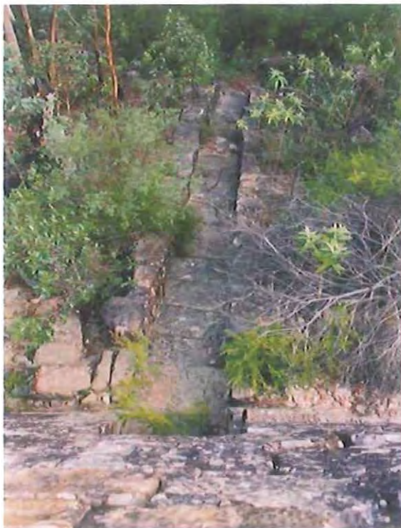
Figure 4-26: Stone culvert in retaining wall, Devine's Hill. (Photo: Ingereth Macfarlane)
