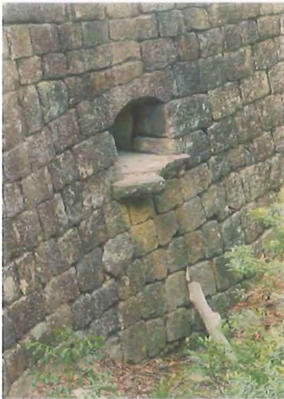
Figure 4-26: Stone culvert in retaining wall, Devine's Hill. (Photo: Ingereth Macfarlane)
