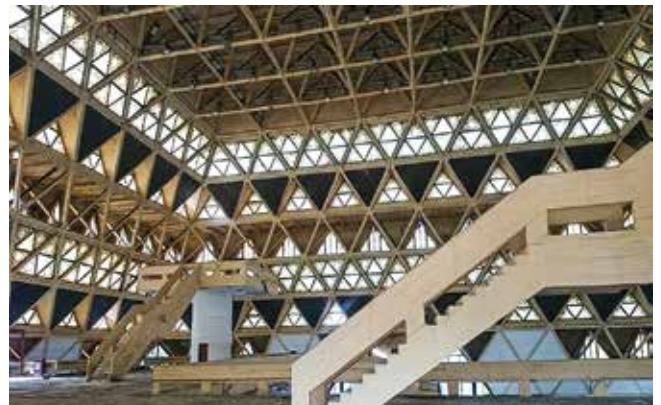
Fig. 7: Interiors of Hall of Nations showing the system of natural lighting, sound state of materials and structure (© Kiran Joshi, September 2016)
