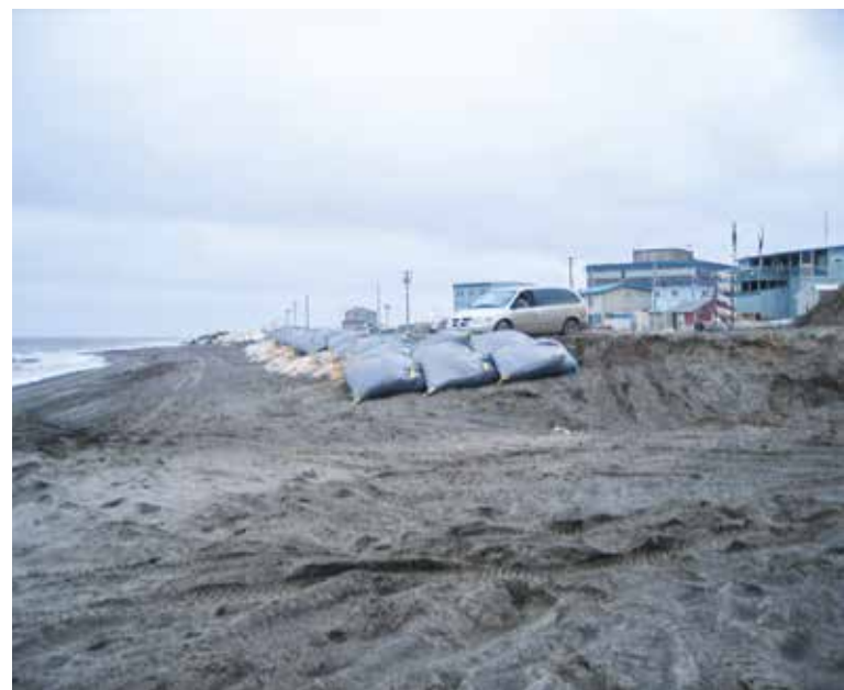
Fig. 2: Attempts to stop coastal erosion in Barrow, Alaska (photo Susan Barr)
