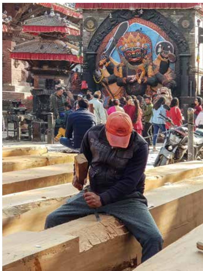
Fig. 2a: Carpenter working on a timber post for the reconstruction of Kasthamandap, with the Kal-Bhairab statue in the background (© ICOMOS Nepal/Kai Weise)
