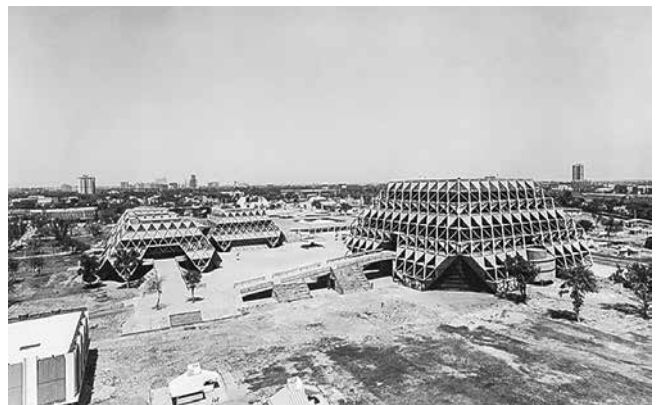
Fig. 1: The Hall of Nations is the largest cast-in-situ concrete space frame structure in the world, exemplifying an economic argument and simple aesthetic of modernity by utilizing minimal resources and indigenous technology in post-Independent India. (© Kiran Joshi, personal collection, September 2016)
