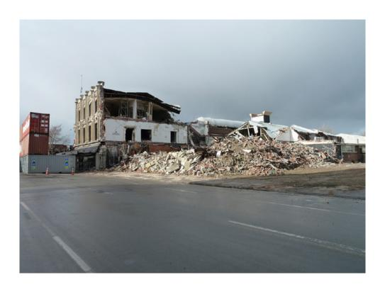
unreinforced masonry (URM) construction. The McKenzie and Willis Building shared party walls with neighbouring buildings, one of which collapsed during the February 2011 earthquake (former A J White building at 232 Tuam Street) (figg. 7 and 8) and another of which was destroyed by fire soon afterwards (Billen's Camping Building, 167-177 High Street).
