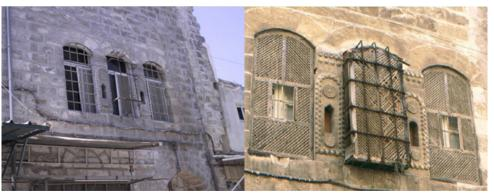
Images, Clockwise from top left: Figg. 74–77. The use of cement mortar and new materials for stabilisation and repair work
