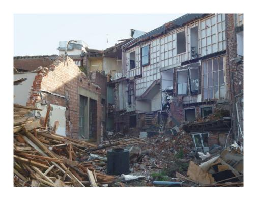
Fig. 8. The unreinforced masonry structures to the rear of the McKenzie and Willis facade have collapsed (Source: Carole-Lynne Kerrigan, n.d.)
