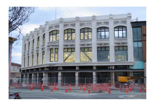
Fig. 15. Restored façade with construction of new building occurring behind. The steel braces supporting are clearly visible through the windows (Source: C. Forbes, 13 September 2016)
