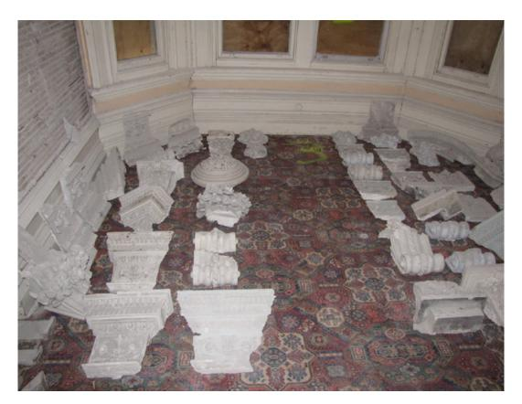
Fig. 30. Plaster brackets have been salvaged, sorted, inventoried and stored for future reinstatement (Source: CCC 25/3/2019)
