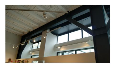
Fig. 20. Detail of steel support structure behind the facade (Source: A. Ohs. 21 November 2019)
