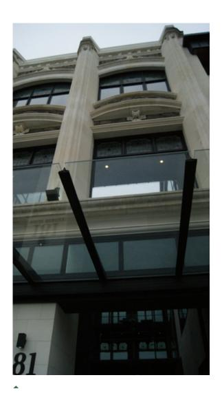
Fig. 19. The new glass awning over the footpath and new shop fronts (Source: A. Ohs, 21 November 2019)
