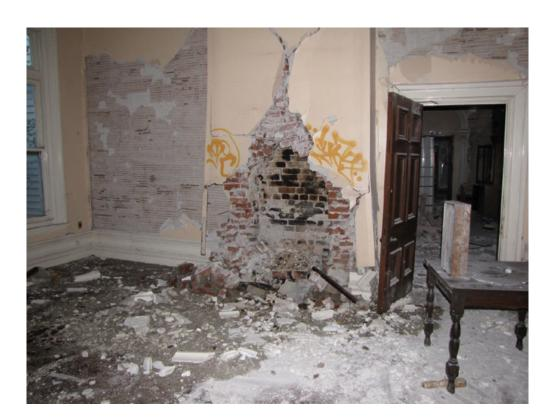
Fig. 25. Brick fireplaces have collapsed (Source: W. Clark, 24/11/2015)
