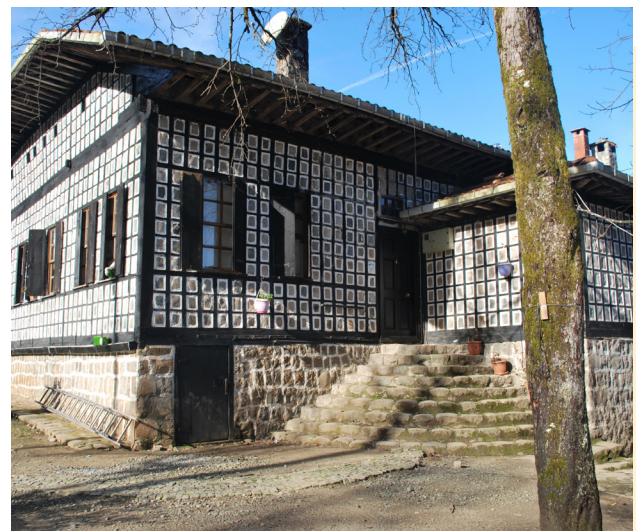
Plate 2 A typical example of stone-infilling technique from the mansion of M.İ. Photo: Gül Aktürk, 10 January 2019.
