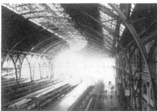
*Here is the interior of the Barcelona rail station. Designed by Andre Montaner, engineer of the « Land and Maritime Machine Building » Company, it was built in 1929 by the « Madrid-Zaragoza-Alicante Railroad Company » (M.Z.A.). It comprises two centerings in the form of a double tri-articulated arch and two lanterns above the naves. These were the last ones built of iron in Europe and were replaced with concrete shelters.*
