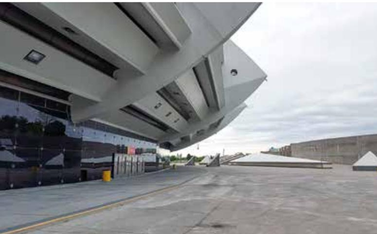
*Fig. 3 The junction between the Stadium and esplanade showing the console structural system, its expressive use of concrete and original glass wall*
