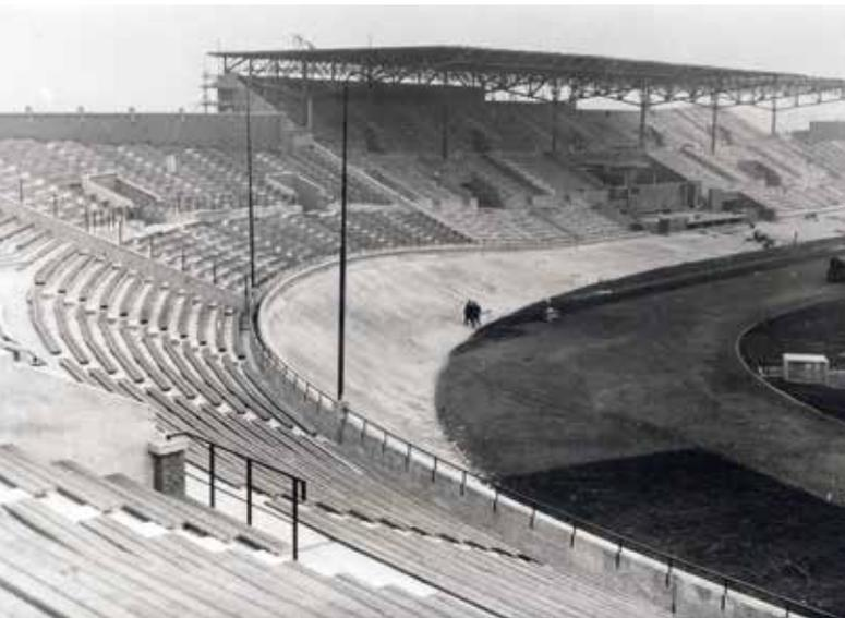
*Fig. 5 The Olympic arena with its concrete framework and cycling ring under construction (1928)*
