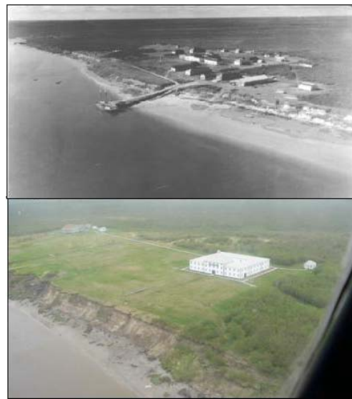
Figure 2. York Factory in 1923 (top) and in 2005. The Depot (centre of bottom photograph) and library (to right) are the only historic buildings left. Only part of the historic site, with more than seventy archaeological features, is kept clear of willows (Photos from National Archives of Canada, K.Skafffeld)
