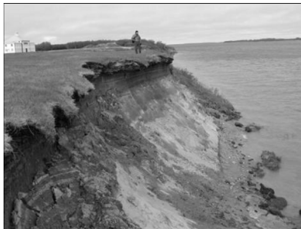
Figure 3. Bank slump, Hayes River at high tide.(photo from K.Skafffeld)
