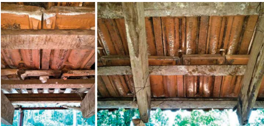
Figure 15. Two, instead of one baton was fixed along the ends of the roof's framework. Figure 16. Two slits of the beetle-nut tree were used as batons
