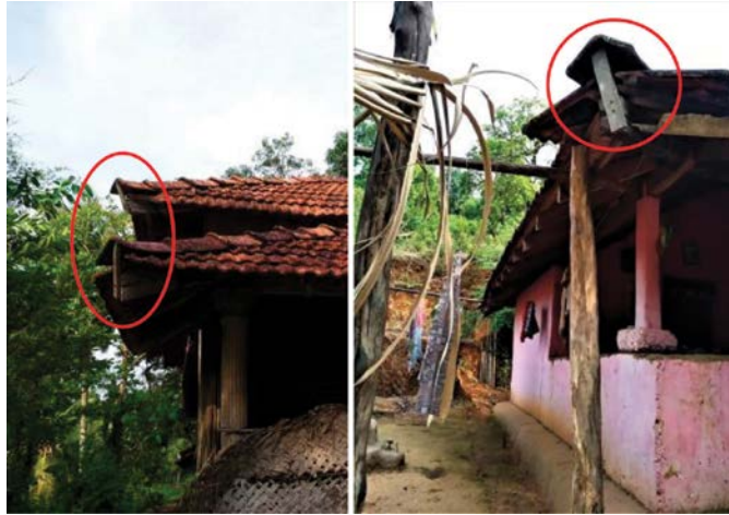
Figure 17 and Figure 18. Small, wooden batons were fixed on roof corners
