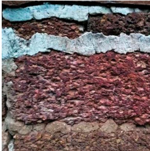
Figure 7. Earthen mortars with lime re-pointing
