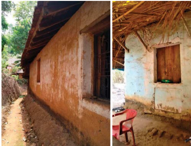
Figure 3. A small, earthen gradient covered the foot of external walls
