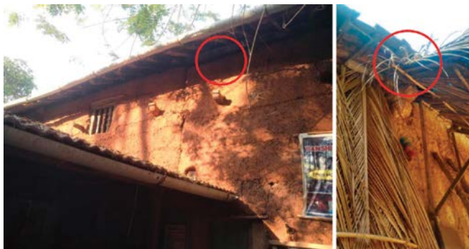
Figure 11. Wooden pegs along the lengths of some façade walls
