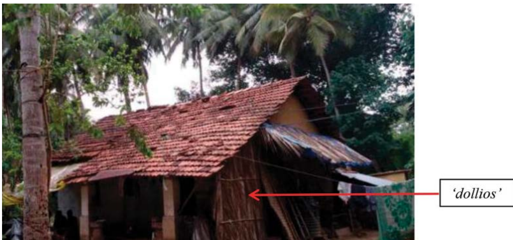
Figure 8. Palm-leaf barriers poised parallel to earthen walls protected walls from rainwater
