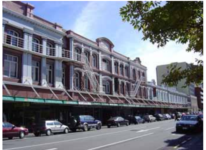
Fig.2 The buildings which make up Cashel Chambers were constructed between 1882-1919, and made a significant contribution to the streetscape setting of Cashel Street and Bedford Row behind.
