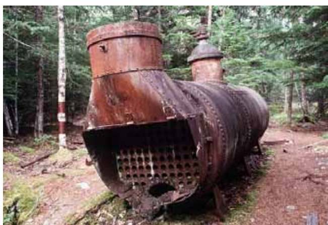
Fig.8 Boiler for train Parks Canada H.10.99.06.01(16)
