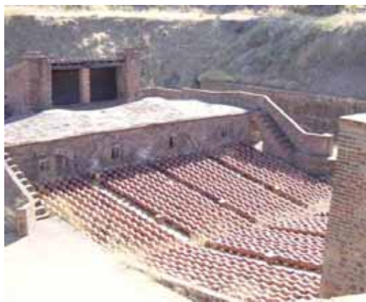
Fig.2 "Aludekses" furnaces in Almaden
