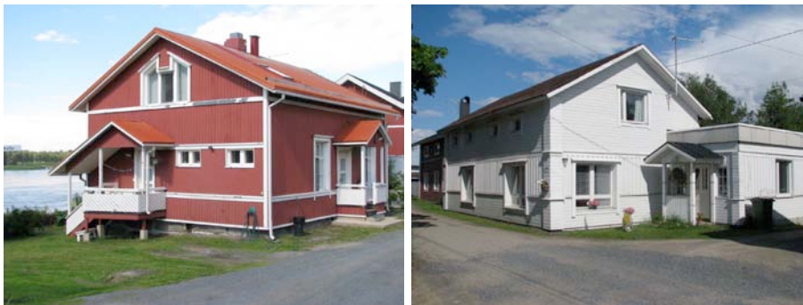
Figure 5 and 6. Typical buildings after alterations: windows have been enlarged, a thick layer of insulation has been added outside the building and the original, simple type of boarding has been changed. (Photos A. Soikkeli)
