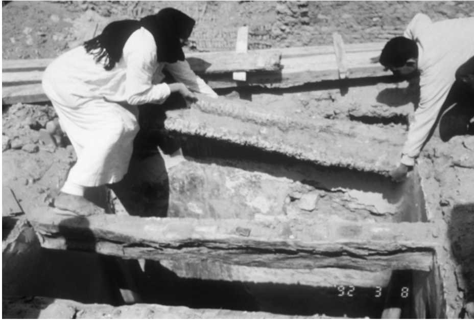
Replacement of the palm beams of the roof over the painting in the Coptic church in Naqlun in the Fajum oasis, Egypt.
