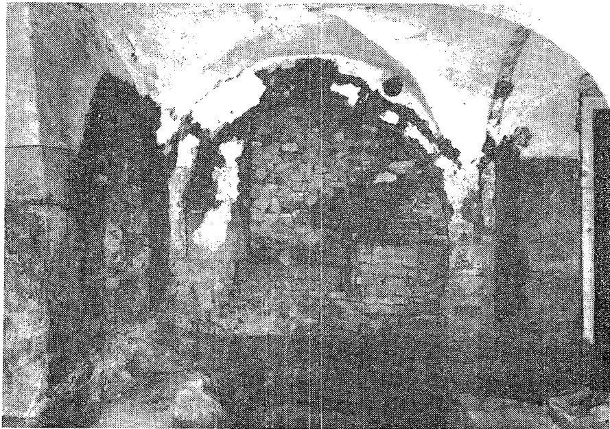
Ground floor, main room. In the background, site of the original oven with its arches. Photo taken during the restoration
