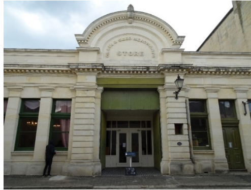
(a) Harbour Street elevation/New parapet
