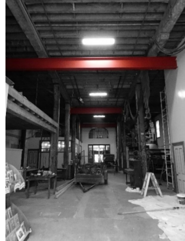
(c) 3 Steel Cross Beams
