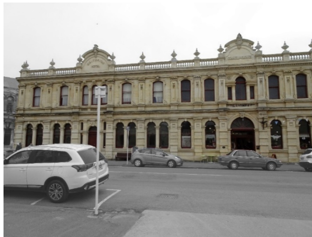
(a) Visible colour variation in Oamaru limestone parapet, indicating recent reconstruction works
