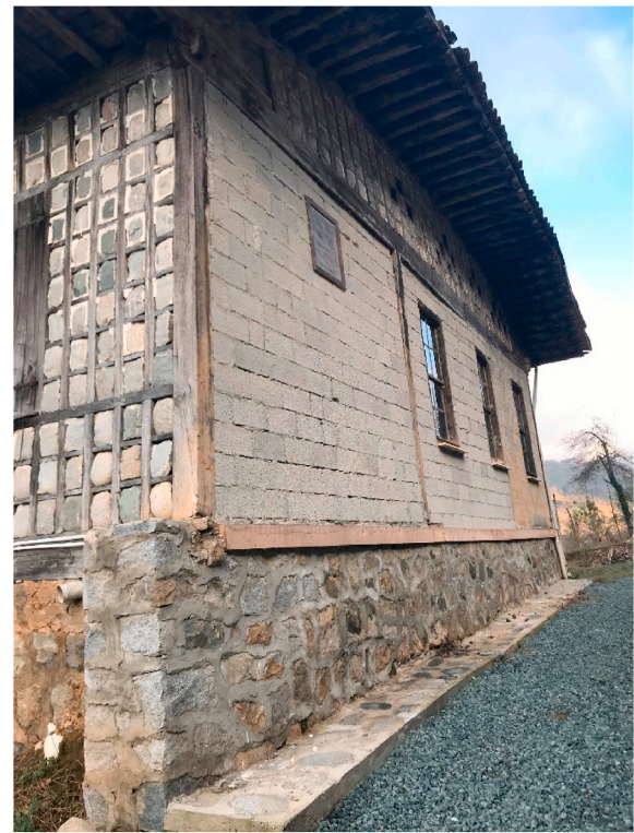
Fig. 9. The degradation of the rear façade of the Şevket Atac House due to landslides in Çağlayan Village in Fındıklı of Rize. The photograph was taken by the first author, Gül Aktürk, on January 12, 2019.
