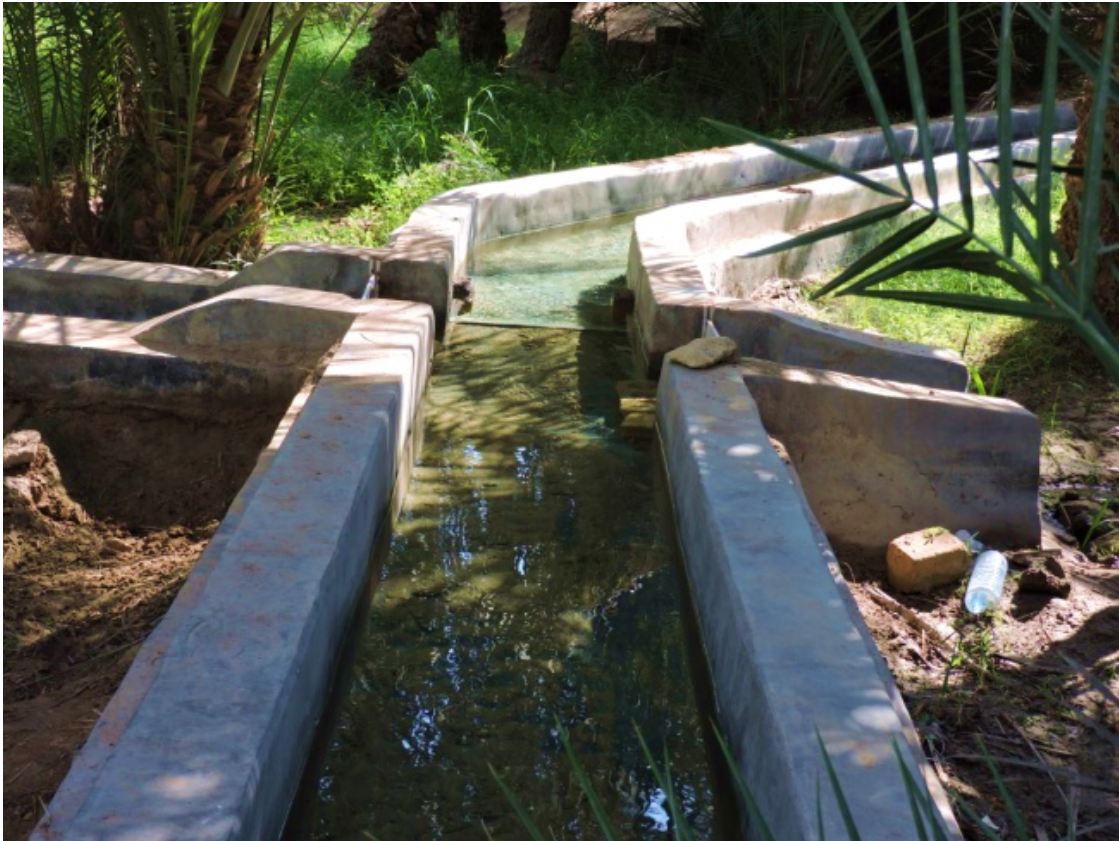
Fig. 10: Cement channels are now used for water distribution (Harrouni, 2018)
