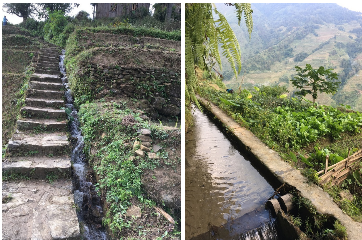
Figs. 12-13: Irrigation system of the rice terraces (Thibault, 2019)
