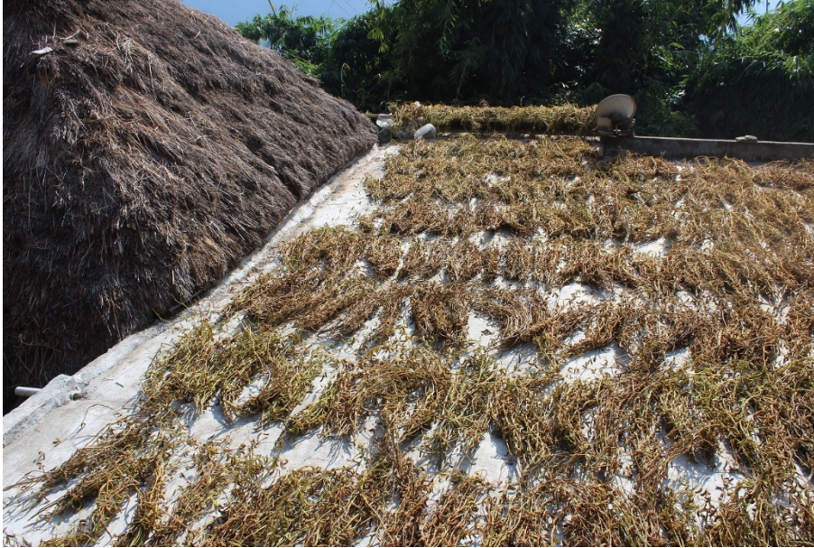
Fig. 6: Flat roof with beans drying (Martin, 2019)
