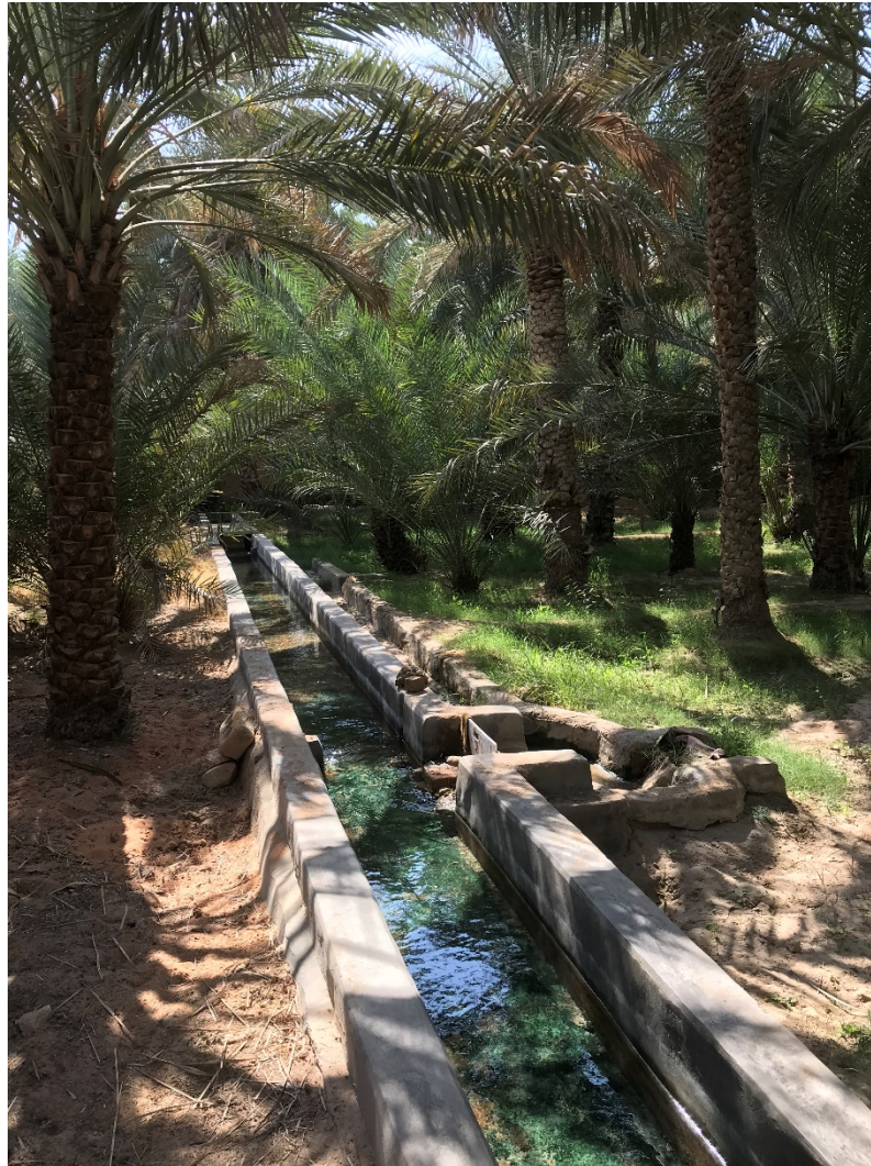
Fig. 4: Ancient technology with modern materials – concrete walls of the tributary channels ( awamid ) and plastic sluices for today's aflaj (Wigboldus, 2018).
