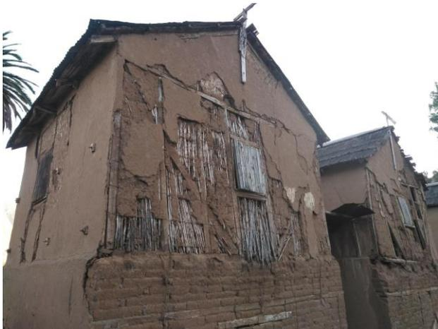
Figure 6. A singular case of ‘quincha’ in Chalinga. The lower area is built with adobe.
