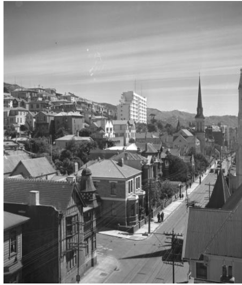
Fig 6 View from the intersection of Ghuznee and Willis Streets looking north along Willis Street, toward St John's Presbyterian Church (on the left) and Dixon Street Flats (centre) 1942, ATL ¼ - 000821
