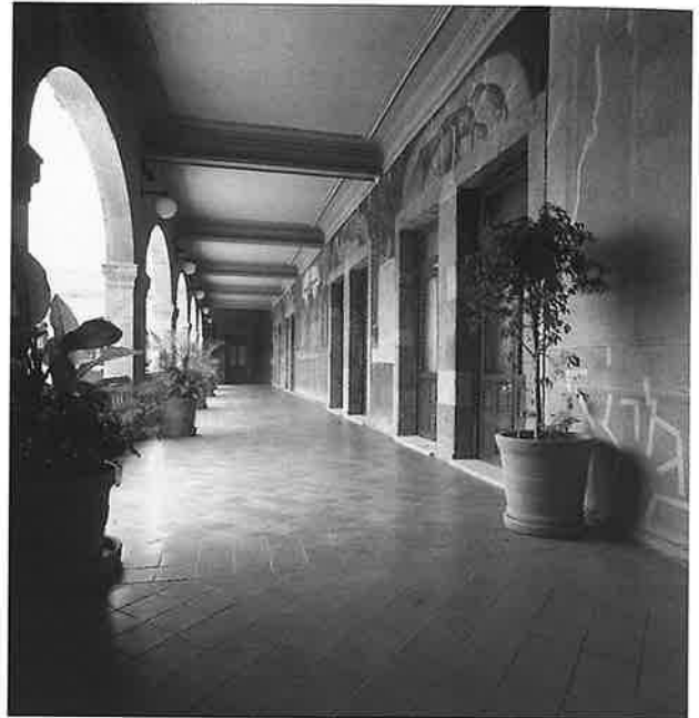
Fig. 8. An upper floor gallery to one of the courtyards of the former Convent of the Incarnation. Photograph by Gabriel Figueroa Flores
