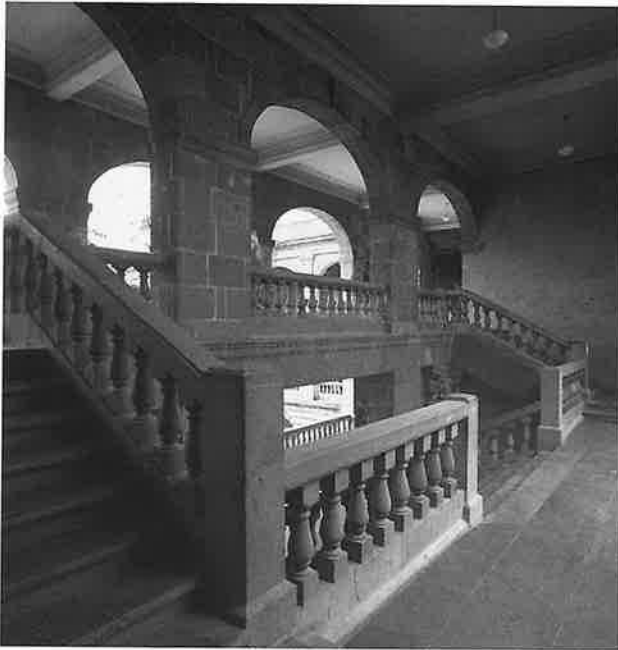
Fig. 7. The grand staircase between the two courtyards of the former Convent of the Incarnation. Photograph by Gabriel Figueroa Flores
