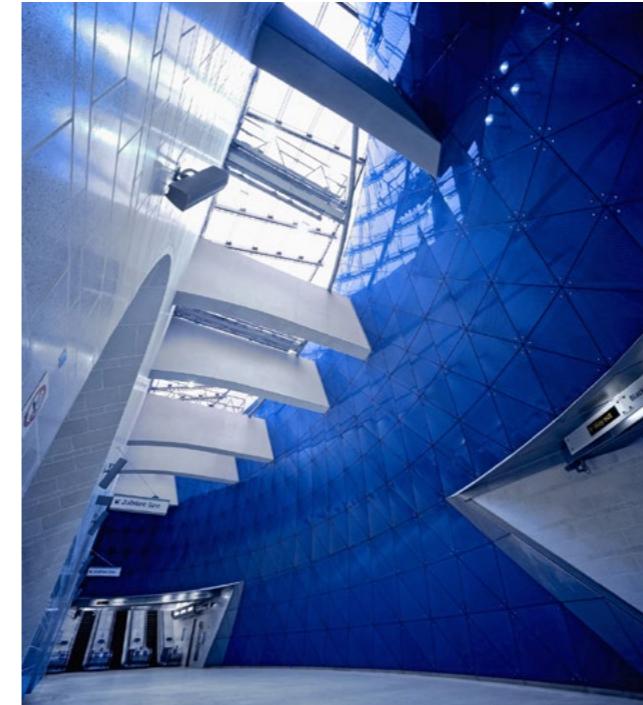
Fig. 3: Southwark underground station, close-up of curved blue glass screen designed by Beleschenko. The tiles are held by stainless steel 'spiders' connected to a steel frame
