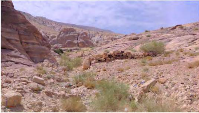
Dam 2 Before re-construction
