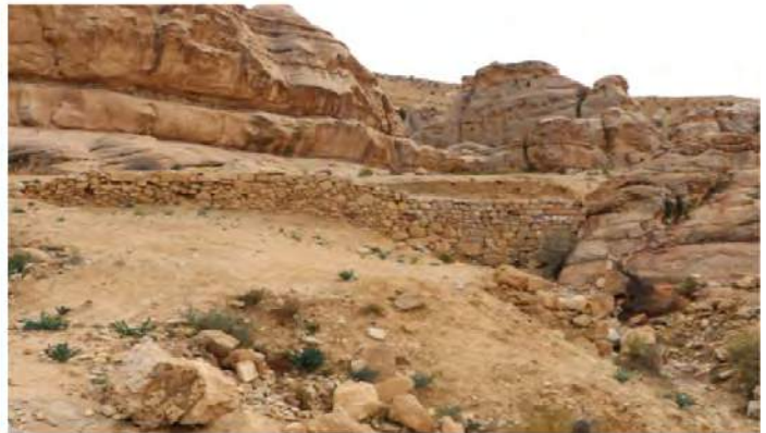
Dam 4 After re-construction
