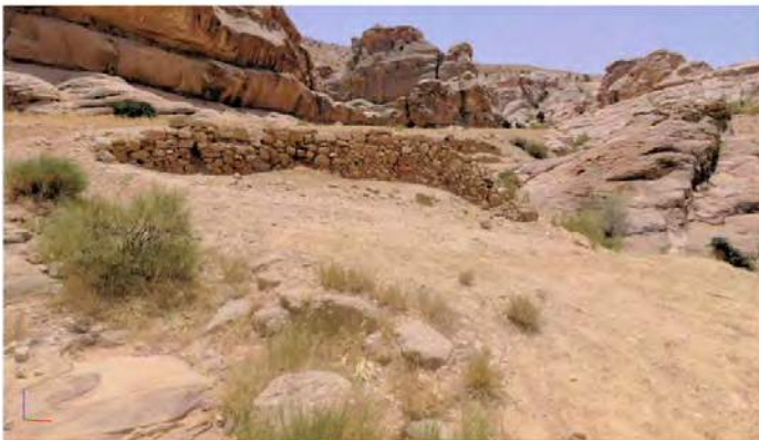
Dam 4 Before re-construction
