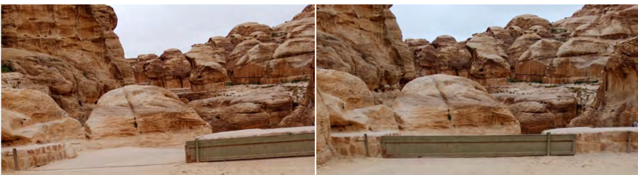
Figure 35: Retractable barrier at the entrance to the Siq, open (left) and closed (right) (Photos: Muhannad Rawadieh, 2024)
