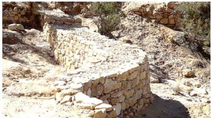
Dam 6 After re-construction
