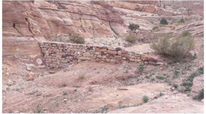
Dam 2 After re-construction
