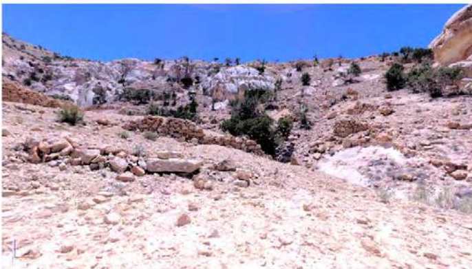
Dam 6 Before re-construction
