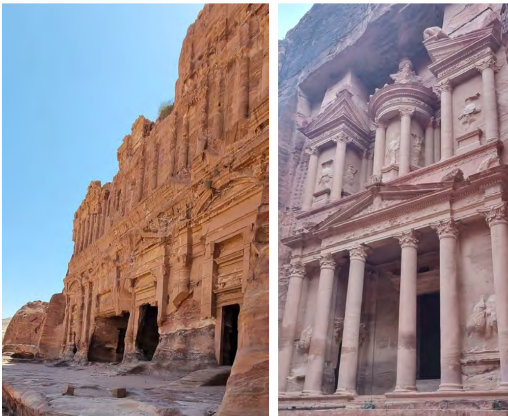
Figure 32: The impact of sandblasting and wind erosion on the Royal Tombs (left) and Al Khazneh (right). Both sites are sensitive to erosion but have different sensitivities (Photos: Taher Falahat, 2022)
