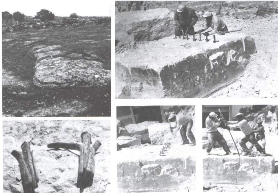
Figure 4 – Working of the Modica stone plates
