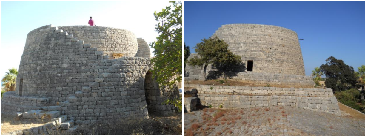
Figure 2 -3 – (on the left) The double-flight-of-stairs system of the muragghio of Villa Trippatore in Sampieri, Ragusa; (on the right) the muragghio and the system of terraces, cisterns, garden in which it lies.
