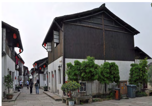
Figure 2. Typical construction of houses in Xiao He Zhi Jie (Peter Phillips)
