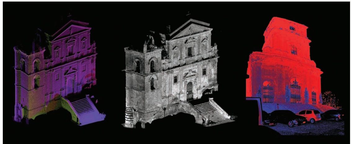
Fig 02) Examples of 3D decay map- ping: the case study of the Ca- thedral of Enna
