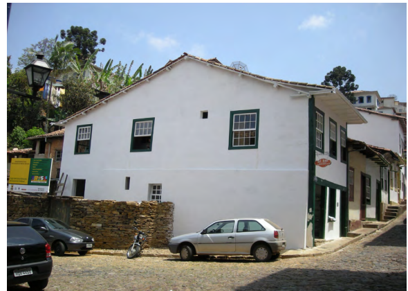
Figure 2. Ouro Preto - MG after recovery
